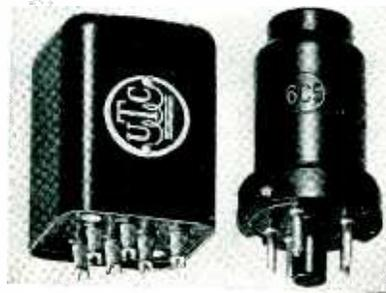
tubes. These units are claimed to have a response plus or minus 2 db. from 30 cycles to 20,000 cycles. They measure 1 7/16 x 1 7/16 x 1 15/16 in., having an average weight of 6 1/2 oz. They are intended primarily for noise meter, aircraft and remote pick-up work.
