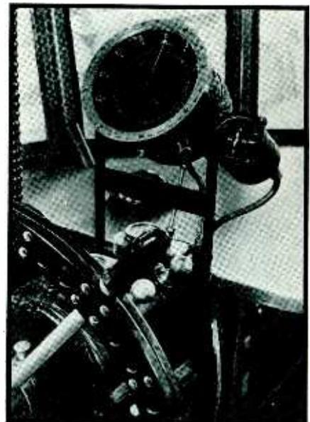
The small indicator is for use with the blind-landing radio beam, for guiding the new zeppelin through fog
