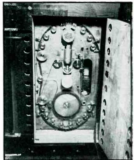
Phototube and film mechanism which delivers advertising messages to the public
