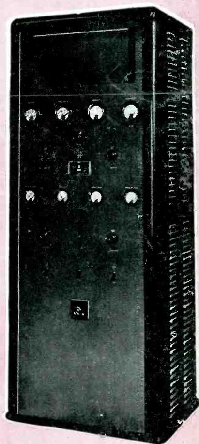
**NEW RCA TRANSMITTER 250-D**...rated at 250 watts and 100/250 watts. A low power transmitter and a basic exciter unit. Simple, efficient operation. Fine performance. Easy accessibility. Low operating cost. Most modern design. 16 operating meters, conveniently located. Interlocking doors for safety. Easy installation.
