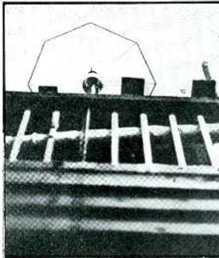
Berlin's "pancake" television radiator, 453 feet high, which sends video images on 6.7 meters. The "edges" of the pancake are horizontal dipole elements which concentrate the energy in the horizontal plane
