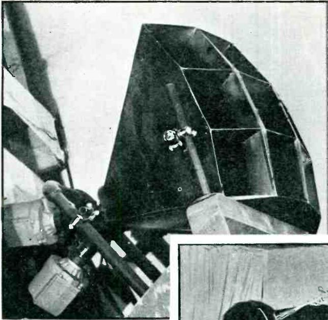
On either side of the stage are semi-circular covers extending upward 80 feet. At the base of each and facing is a group of 4 loud speakers. Sound strikes these deflecting covers, reaches the audience indirectly, providing reverberation. Below—
