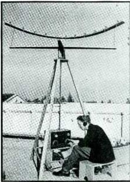
Parabolic reflector antenna used for receiving 1.5 meter signals from a stratosphere explorer balloon. At receiver is Prof. Easton of Caltech
