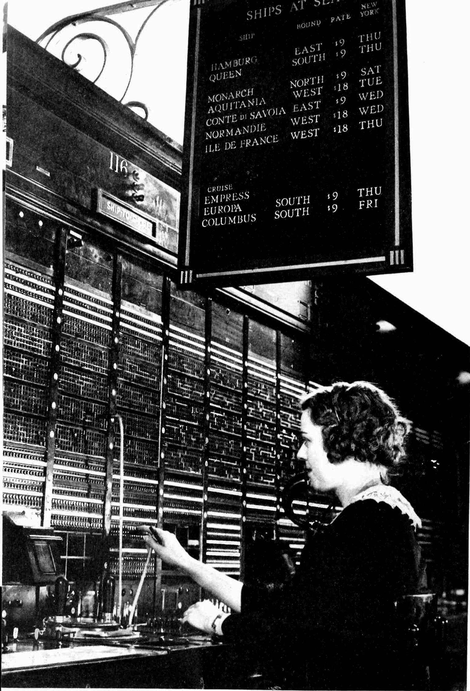
Toll operator putting through ship-to-shore call at 32 Walker St., New York City, from which position connection can be made with 34,000,000 telephones in 68 countries
