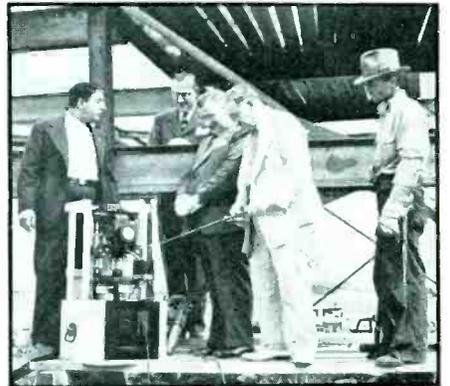
A portable transmitter, with an induction heating coil attached in place of the antenna, was used to heat the last rivet in the steel work of the RCA Exhibit Building at the New York World's Fair Grounds. The rivet, suspended in the induction coil, became white hot in less than a minute.
