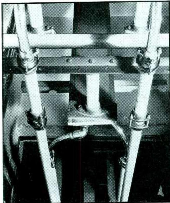
Fig. 3—Method of making bends with copper tubing and bronze fittings
