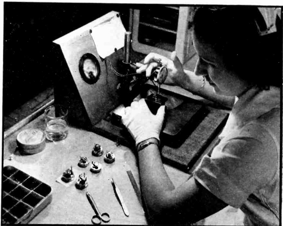
Focus of electron beams in X-ray tubes depends upon placement of filament in slot in focussing cup. In these Westinghouse units the accuracy of measurement is one ten thousandth of an inch
