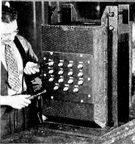
Illustrated above is a 20 KVA, single phase, air cooled transformer built for the laboratory of a large industrial concern. Primary—220/230/240 volts, 60 cycles, and a secondary winding with 22 taps. From 2 to 14 volts in 2 volt steps at 200 amperes, and from 70 to 280 volts in 15 volt steps each at 20 KVA. Below at right is a tiny, compact audio transformer with an exceptionally flat frequency response curve. Designed for light portable audio equipment.
