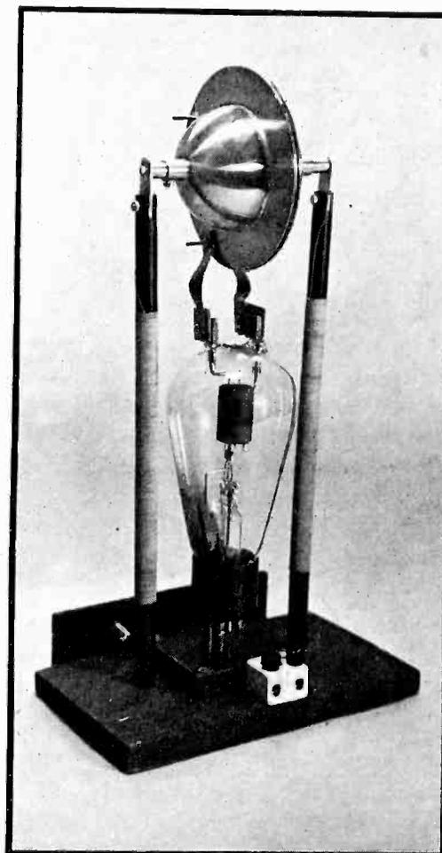
Fig. 3a—Single tube transmitter with RCA 834
