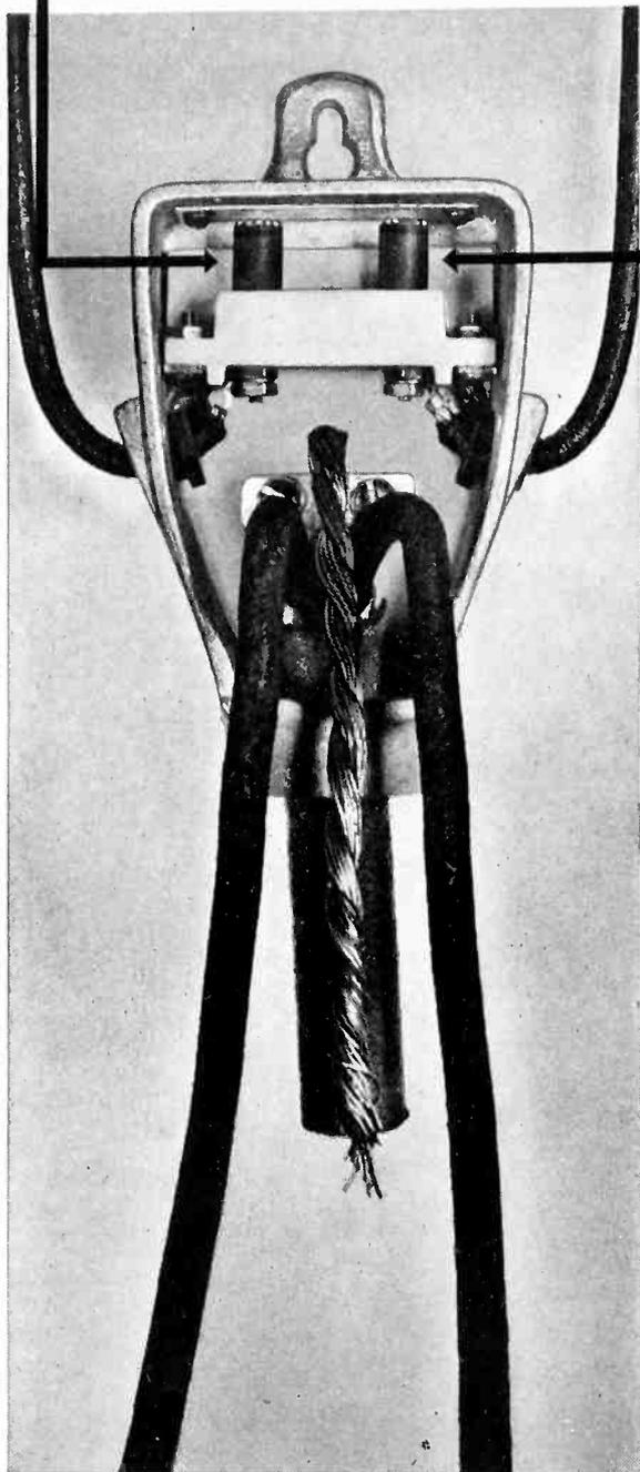
● New M&W Watt-Hour Protector protects meters from current surges caused by lightning or high voltages. It is a low point in the meter circuit; by means of Globar Brand Resistors excess current is shunted to ground instead of passing through the meter.
