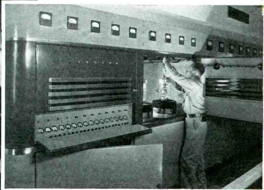
Streamlined front of the new 50,000-watt Westinghouse transmitter at KDKA. Air-cooled tube in the modulator unit being connected at the front panel of the transmitter.
