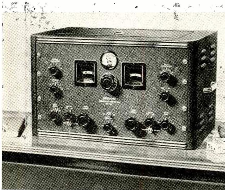
The new and improved Hammarlund Super-Pro Receiver. New features include a variable-selectivity crystal filter, a noise limiter and an "S" meter
