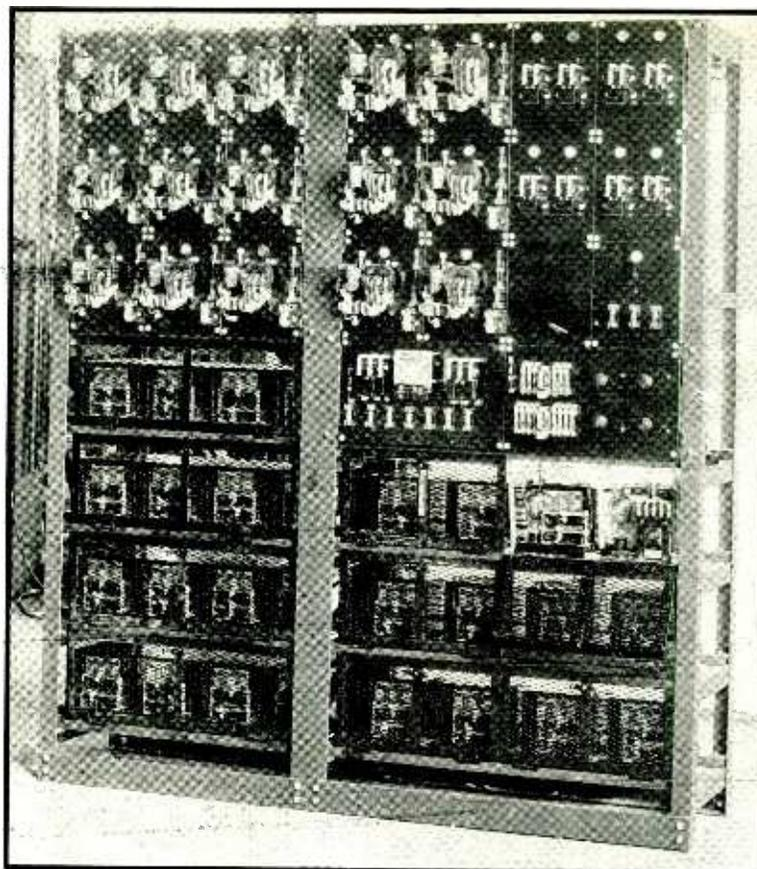
An application of relays for controlling heavy lamp loads, an electronic "Hysteresis" dimmer panel. The heavy-duty contactors at the left are fitted with de-ionization chambers for dissipating the arc
