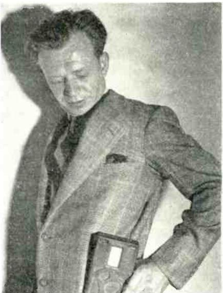
Gilbert Brown, of Hollywood, demonstrating how the four-tube radio which he built, can be carried in the pocket of a business suit. The miniature receiver is 6¼ inches long, 3¾ inches wide, 1¾ inches deep and weighs 1½ lbs. It is equipped with antenna and batteries sufficient for 100 hours of operation
