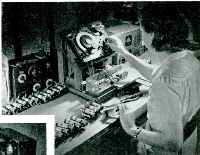
**2** On arrival at the factory, all components are inspected and checked against the laboratory specifications
