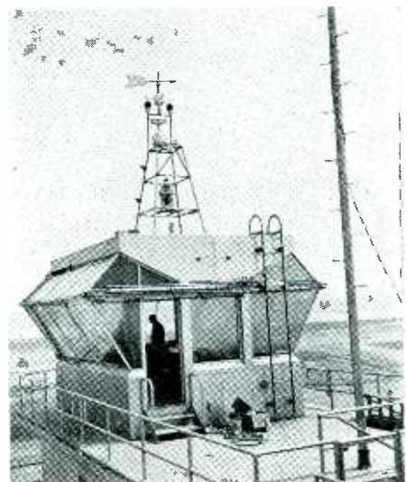
The glass enclosed tower atop the airport building at Washington, D. C., provides an angle of view of 360 degrees for directing the traffic of planes into and out of Washington. The station is also used as a local weather bureau
