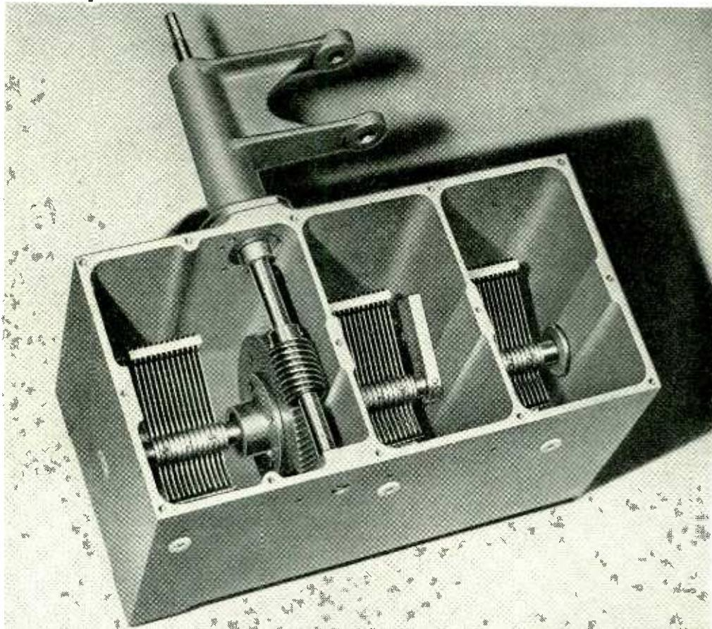
Marine condenser built to withstand severe vibration.
