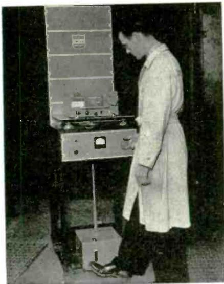
This is United Air Lines' newly-designed vibration generator for testing aircraft radio equipment under conditions considerably in excess of those encountered in flight. H. N. Wilcox, who developed the device, is putting a radio receiver through a typical test. An air-operated generating unit (below) actuates the test table to which the radio set is attached (above)
