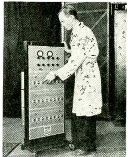
This signal generator is used for aligning the numerous circuits of all aircraft radio receivers carried aboard United Air Lines' Mainliners. E. A. Jensen, who designed the equipment, is operating the push buttons which permit the selection of any of 24 crystal controlled frequencies
