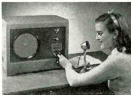
A new Western Electric magnetic recording device is now being used by many as an aid to speech improvement. The subject's speech is recorded magnetically on a steel tape. By turning the switch immediate playback is possible, which enables the detection and correction of errors of pronunciation, emphasis, or tone. As it records, the mirrophone automatically erases or demagnetizes previous recordings
