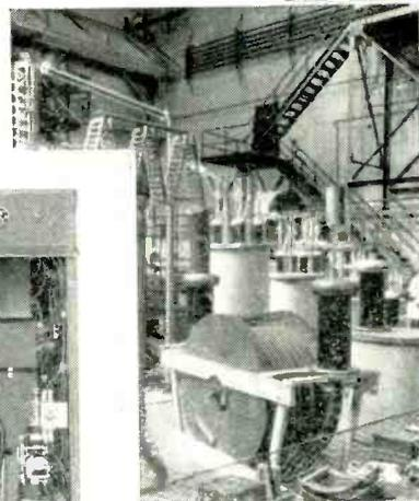
**RECOVERING VALUABLE PARTICLES** from flue gases in smelters, sulphuric-acid plants, cement mills, plants for detarring natural gases, etc. In many applications, as in the fly-ash precipitator above, precipitators powered by kenotrons are used to remove solid particles from factory smoke which would otherwise be deposited over the surrounding country.
