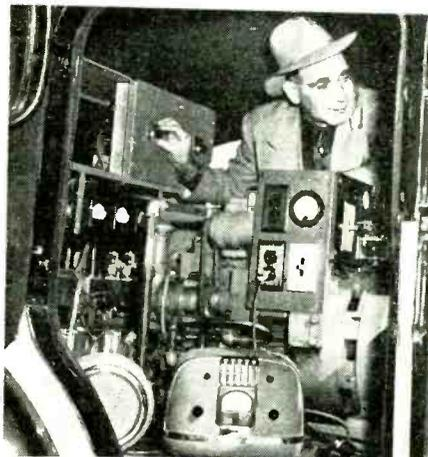
Mobile radio equipment installed in a powerful automobile is operated by a gasoline motor which also generates electricity and enables the police department to broadcast and receive messages in any emergency
