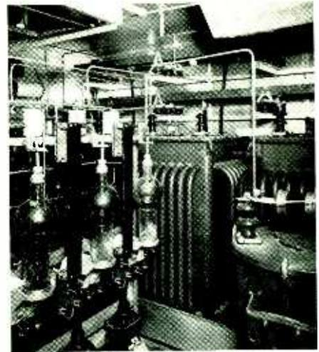
High-vacuum tubes and associated mercury-arc rectifiers comprising part of the equipment in the plywood manufacturing plant's balcony. The equipment turns out 400 kw of r-f at approximately 2000 kc
