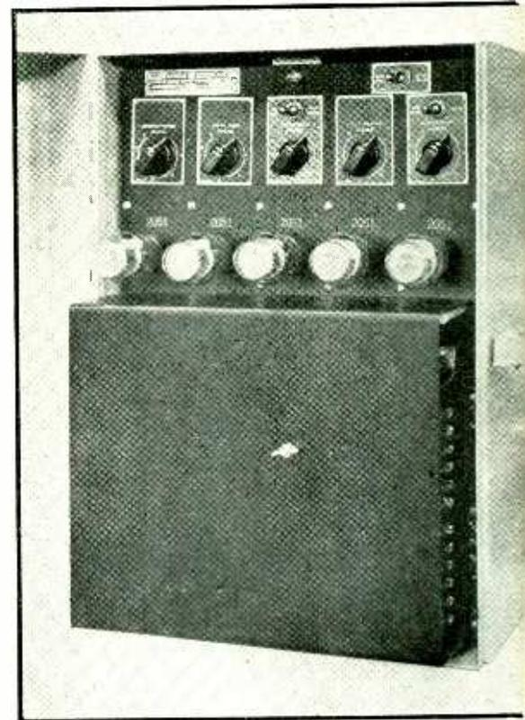
Typical electronic sequence timer of the 9B type, designed for use with welding power control units of the synchronous variety
