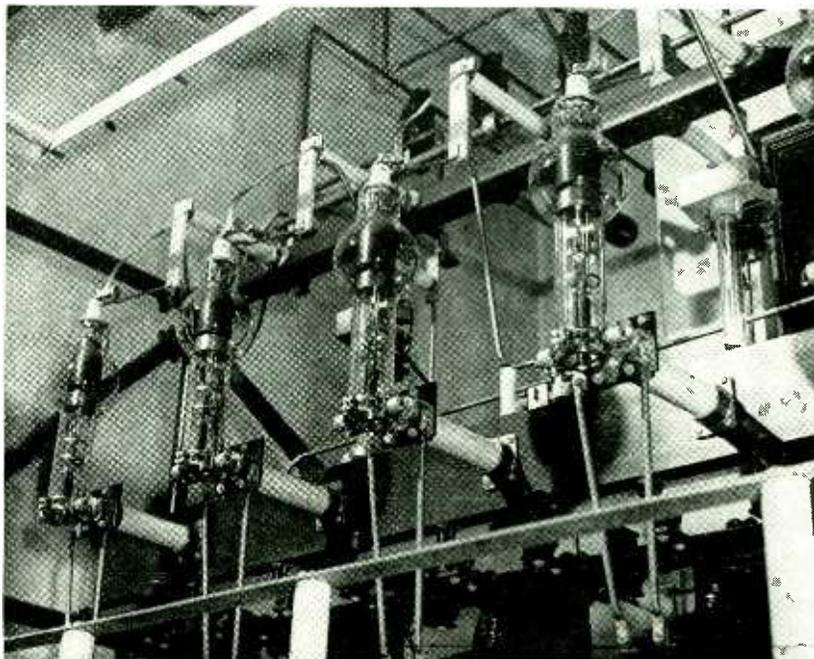
These rectifier tubes supply d-c power at 18,000 volts to operate the 50-kw transmitter of station WHN at East Rutherford, N. J. This station serves the New York City metropolitan area
