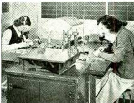
Sodium light is being used in several important war plants for surface inspection by microscope, because of its efficiency in the detection of pits, cracks, and flaws in materials. The sodium lamp is essentially an arc lamp, and differs from the incandescent in that it requires a special socket and individual control for each lamp. The unusual perception of detail under sodium illumination is due to the monochromatic nature of the light
