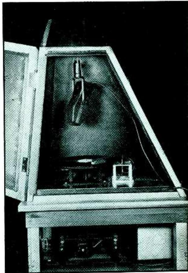
Fig. 9—An internal view of the chamber used to measure the response of record noise
