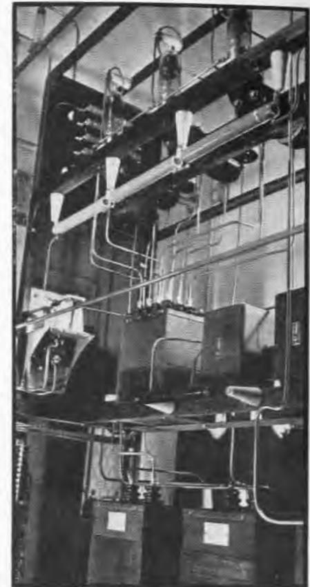
This open-side power frame, in the screened enclosure behind the cabinets, supports main and buffer rectifier parts
