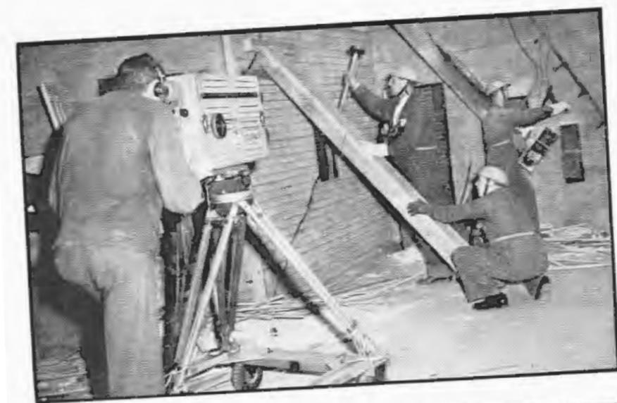
**DEMOLITION**—Experts show distant defense workers how best to prop up a shaky wall and handle dangerous trailing electric wires
