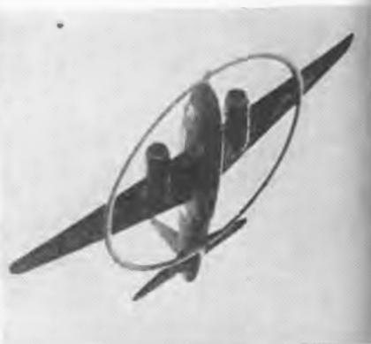
The minesweepers of the air are equipped with a hoop-shaped casing extending all around them and secured to their nose, wings and tail. The casing holds a magnetic coil and current is supplied by an auxiliary engine. This equipment was designed to set up a magnetic current which would set off the mine. The crews are severely jolted when the mines are exploded
