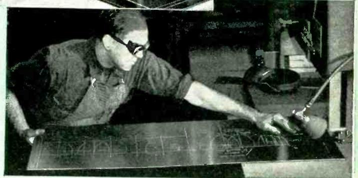
After checking the steel plate against the original drawing, it is cut to shape. The entire process, from drawing to templet is completed in only one hour.
