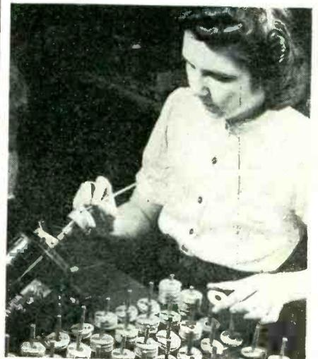
Applying colloidal graphite solution (Aquadag) to discs for copper-oxide rectifiers with a brush while the discs are rotated by an electric motor at a Westinghouse plant. The solution reduces contact resistance
