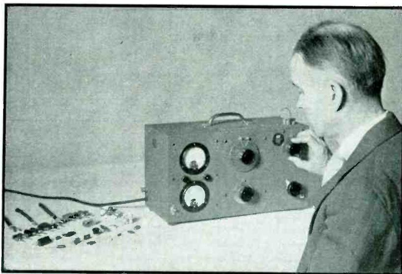
Q-meter used in VHF investigations of radio components covered in this article
