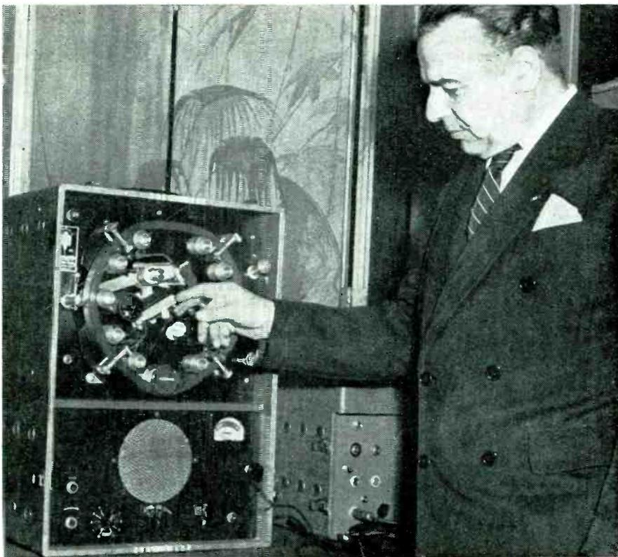
Jay Fonda adjusts the embossing stylus of the cellophane tape recorder he developed. The machine records eight hours of sound on a 350-foot endless cellophane ribbon one-inch wide
