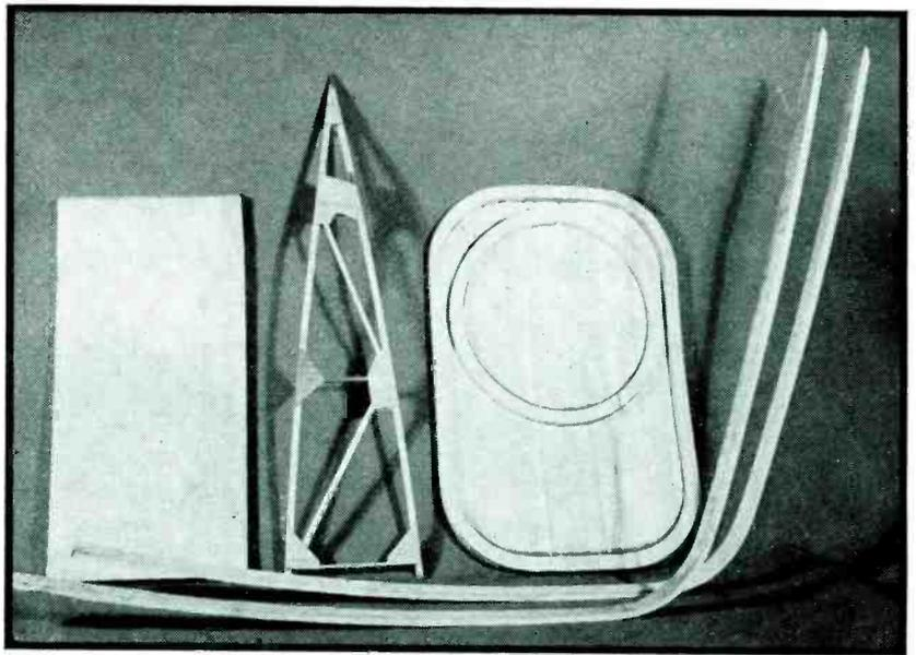
FIG. 4—Some aircraft parts made by the use of r-f heating. Left to right: curved-laminated stock for fuselage reinforcing; wing rib web; bomber door; sections of fuselage ring
