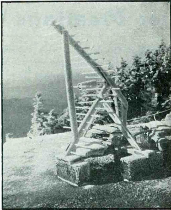
Square-corner antenna originally used at Clingman's Peak to receive 337-Mc signals from the 25-watt Winston-Salem relay transmitter W4XGG
