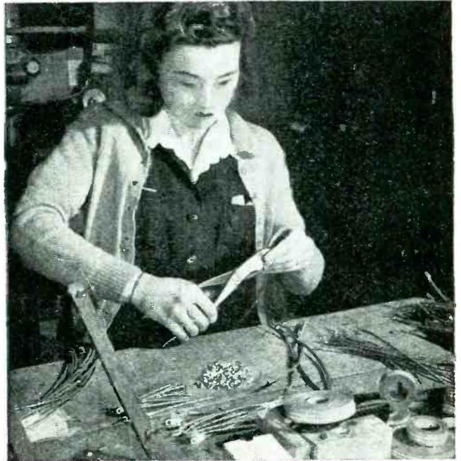
Inexperienced operators can make perfect Indent connections right from the start, and from three to ten times faster than by the older soldering methods. Absence of acid, which frequently causes finger burns, also makes job cleaner and faster.
