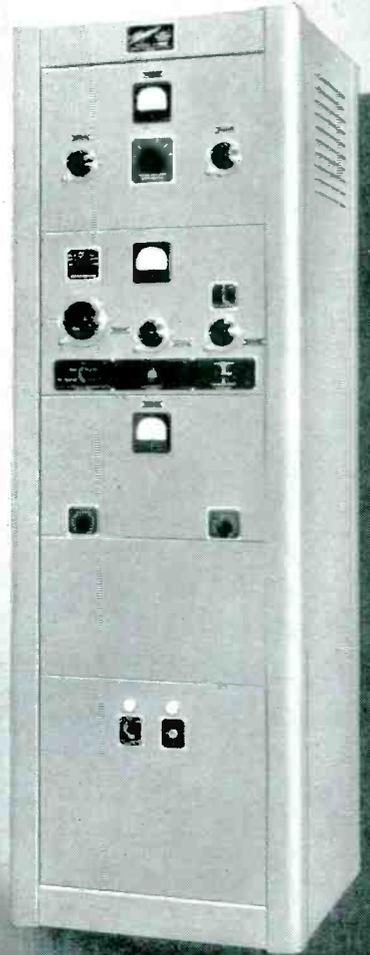
TEMCO Model 252-GSC, 200 watts output, A1, A2, A3 emission; frequency range 2 to 16 megacycles, with provision for 4 crystal controlled frequencies and electron coupled master oscillator.
