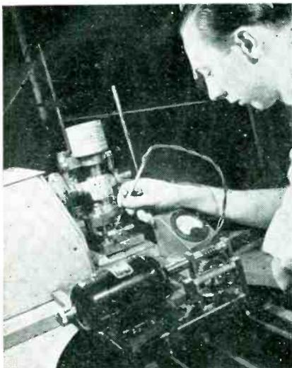
An operator checks the temperature of a hydrogen flame used in conjunction with a punch press to form glass jewels for meters. The glass rod is fed into the press by the motor drive in the foreground
