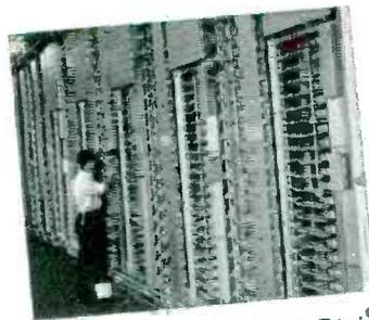
★ Federal's Telephone Division also manufactures, for export and other uses, automatic central office telephone equipment, automatic private and private branch exchange switchboards, telephones and a complete range of telephone equipment.
