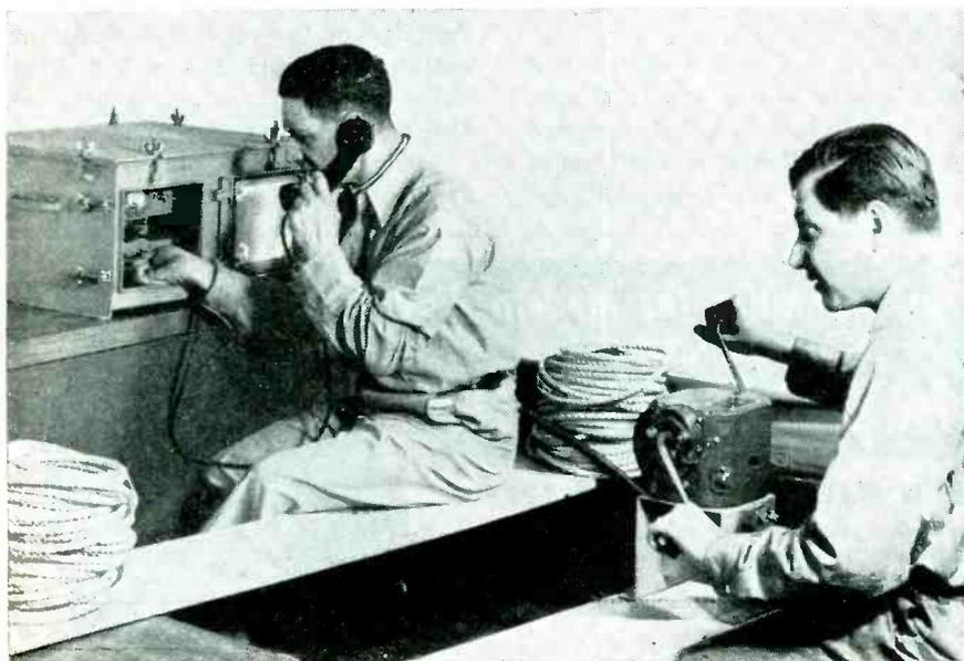
A combination radio-telegraph-telephone set for use in life boats is demonstrated by employees of Radiomarine Corp. of America. While one man cranks the generator, the other operates the equipment to contact nearby ships
