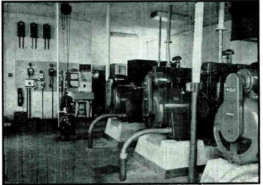
Generating plant at WMIT transmitter site, Clingman's Peak. Three diesel-electric sets generating 75 kw apiece are used
