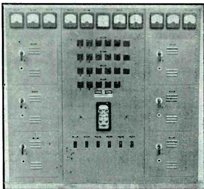
Power-control switchboard at the transmitter site. It permits remote control of the station's generators
