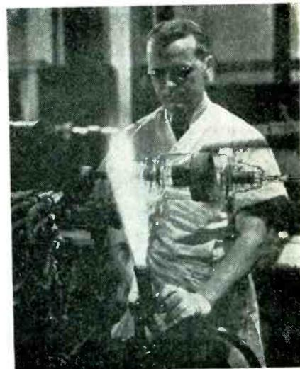
The photo shows a 400-watt vacuum tube being annealed after the filament mount is sealed. The tube is rapidly rotated in a glass lathe during annealing to remove internal strains that may be set up in the glass during sealing. Jens Aakjer, glass craftsman, adjusts the torch used for heating the glass at the Westinghouse Lamp Division, Bloomfield, N. J.
