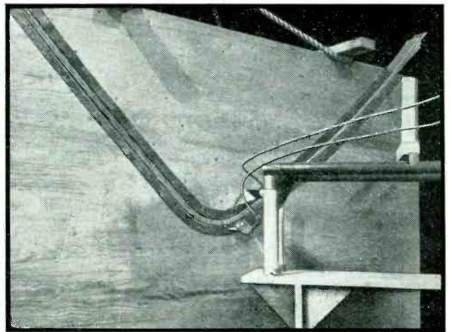
FIG. 9—The forms shown in Fig. 8 with the load in place. Eight sets of hand-clamps are used to obtain pressure
