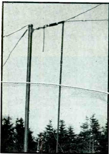
Close-up of the receiving rhombic, showing the feed-line end at which the quarter-wave transformer section encased in a copper pipe and the concentric line discussed in the text are used
