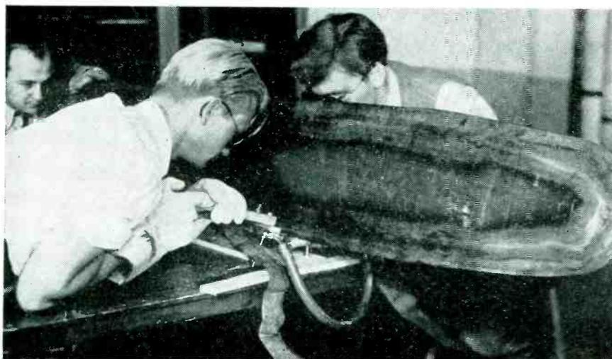
Technicians braze a fillet along the inner edge of a hollow propeller by induction electronic heating in the Westinghouse high-frequency laboratory
