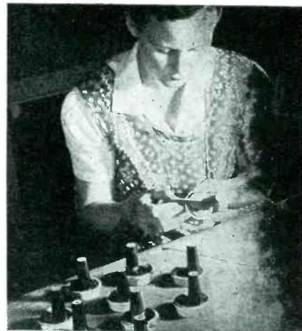
Checking dimensions of Prestite insulator used for terminal posts on capacitors for aircraft equipment to prevent flashover at high altitudes. The insulator, a Westinghouse product, holds up at altitudes of 60,000 feet and resists temperature changes from 234 deg. above zero to 15 deg. below. The insulating material is a mixture of clay, feldspar, and flint and can be solder-sealed to metal shield cans
