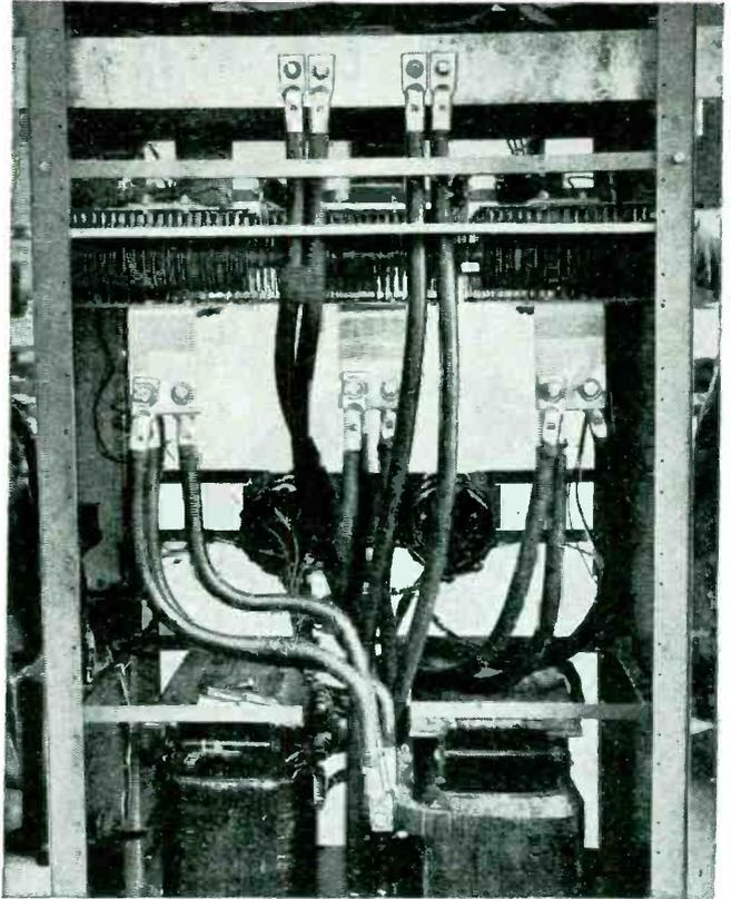
On this large rectifier unit all connections are of the permanent indent type. View shows only terminals; but Indent connectors are also available for end-to-end as well as detachable connections.
