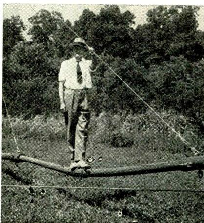
Lightness and strength of the tubular plywood mast are demonstrated by a workman at the plant of Maryland Engineering Co., manufacturers of the mast
