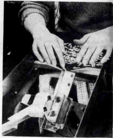
Small assemblies being fed onto a slide for electronic sorting. The chutes for oversize and correct-size assemblies are located at lower left. Units that are too small travel the full length of the slide
