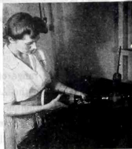
After soaking in warm water for 18 hours, cathode-ray tube bases are inserted in the holder shown above and the tube twisted against the torque of the weight on the arm. Virginia Connick tests the cement on the tube base in this manner at the Dobbs Ferry plant of North American Phillips
