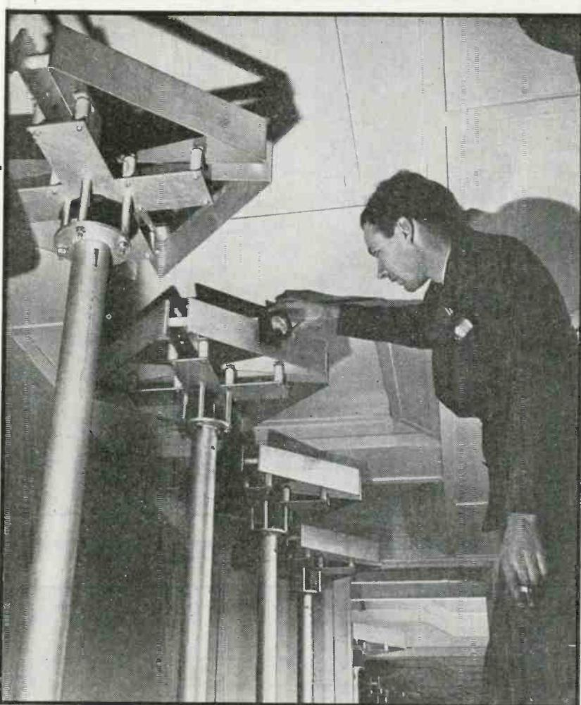
Checking adjustment of loop antenna system for runway localizer of newly-adopted CAA radio instrument landing system
