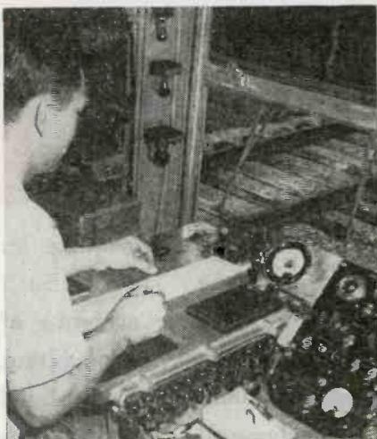
Tape in the recording unit of the rail-fissure detector is watched by a technician as the special electronically equipped car moves along the railroad tracks.
