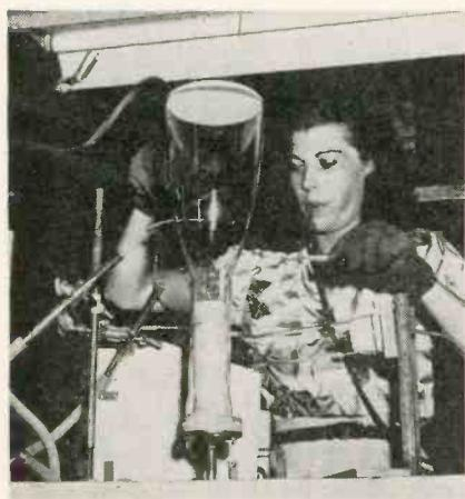
Metallic buttons are sealed-in on cathode-ray tubes at the Dobbs Ferry plant of North American Phillips. The operator controls the air pressure in the tube with her mouth while the gas burner is rotated around the button.
