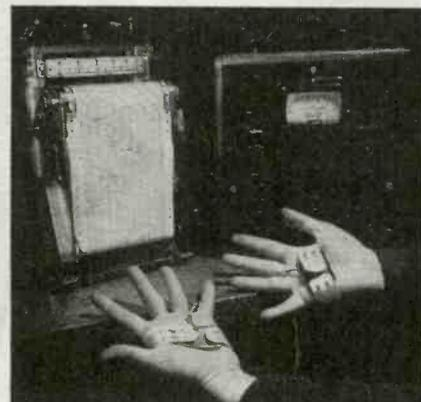
These simple metal electrodes, held in the palms by straps, are the only connection to the subject during a deception test with the Fordham Pathometer
