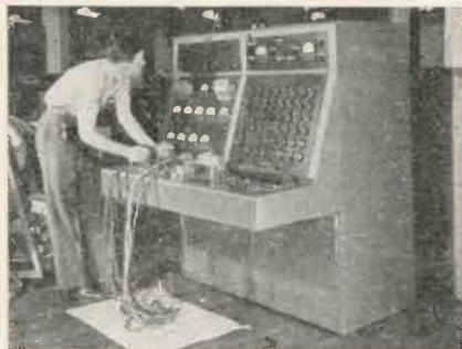
Above is the front view of the Universal Test Unit that preheats all tubes except rectifier, short tests all tubes (each element separately), noise tests RF and AF tests, static tests all tubes for all characteristics except plate resistance and amplification factor, dynamic tests mutual conductance, gain and power output at 400 cycles.
