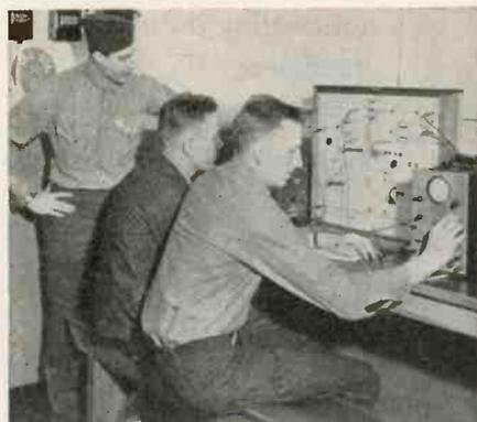
Students use test equipment to study circuit operation. In this instance they are observing wave shapes throughout a d-c amplifier
