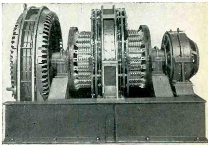
*Motor-generating set made by Hanson-Van Winkle Munning Co., utilizes Mica in the commutators, Micanite V-rings, Empire cloth and tape, for dependable insulation. The twin-commutator generator is rated 20,000 amperes, 9 volts.*
