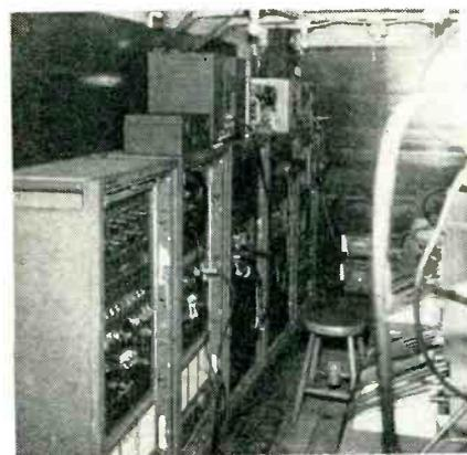
Operating setup of the AN/TRC-6 ppm multi-channel relay station for frequencies between 4,300 and 4,900 mc—
