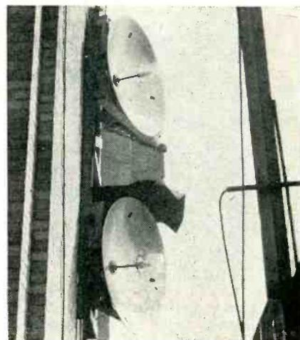
Antennas for receiving and transmitting ptm signals on 1200 megacycles are installed on the IT&T Corp. building at 67 Broad Street, New York City
