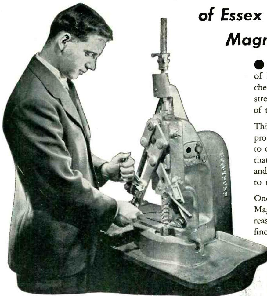
● Before it leaves the plant, every spool of Essex Magnet Wire, #10 and finer, is checked with the *snap test*—a sudden, rapid stretch or elongation to the breaking point of the copper.
