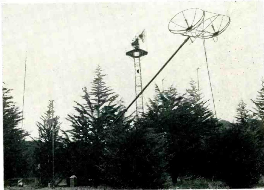
Transmitting and receiving antennas of the Army radio set AN/TRC-5, the 1,400-mc multi-channel equipment using pulse-position modulation, are raised with the help of a jury mast. The 4,900-mc antennas of the AN/TRC-6 ppm set appear at center.—
