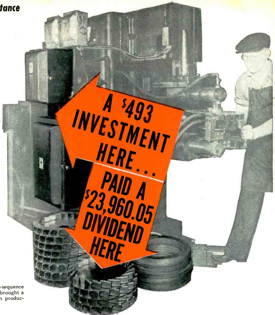
Weld-O-Trol and weld-and-sequence timer added to this welder brought a net saving of \$23,960.05 in production of blower units.
