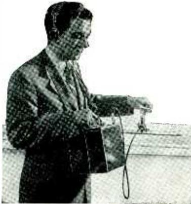
cable. Earphones enable the operator to determine when the two oscillators are set to the same frequency. The entire instrument weighs approximately 11 lb, and may be used as a portable field instrument or on a laboratory bench.
