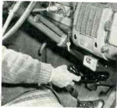
Slide-out type telephone set being used in St. Louis mobile radiotelephone system. Operation is in the 152-162 mc band, with a 250-watt central transmitting station and a 20-watt transmitter in each vehicle. Fixed receiving stations are located in various sections of the city for reliable pickup of the low-power mobile transmitters
