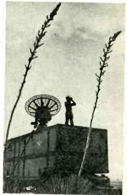
Ground radar used for tracking V-2 rockets in flight
