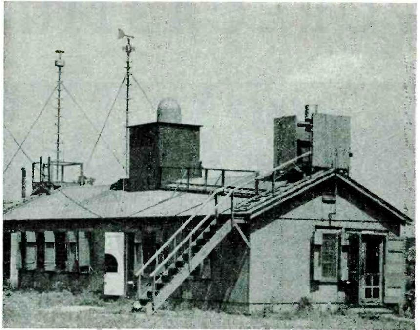
Radar installation in Army weather station for storm detection. Antenna is in radome on roof near center of building
