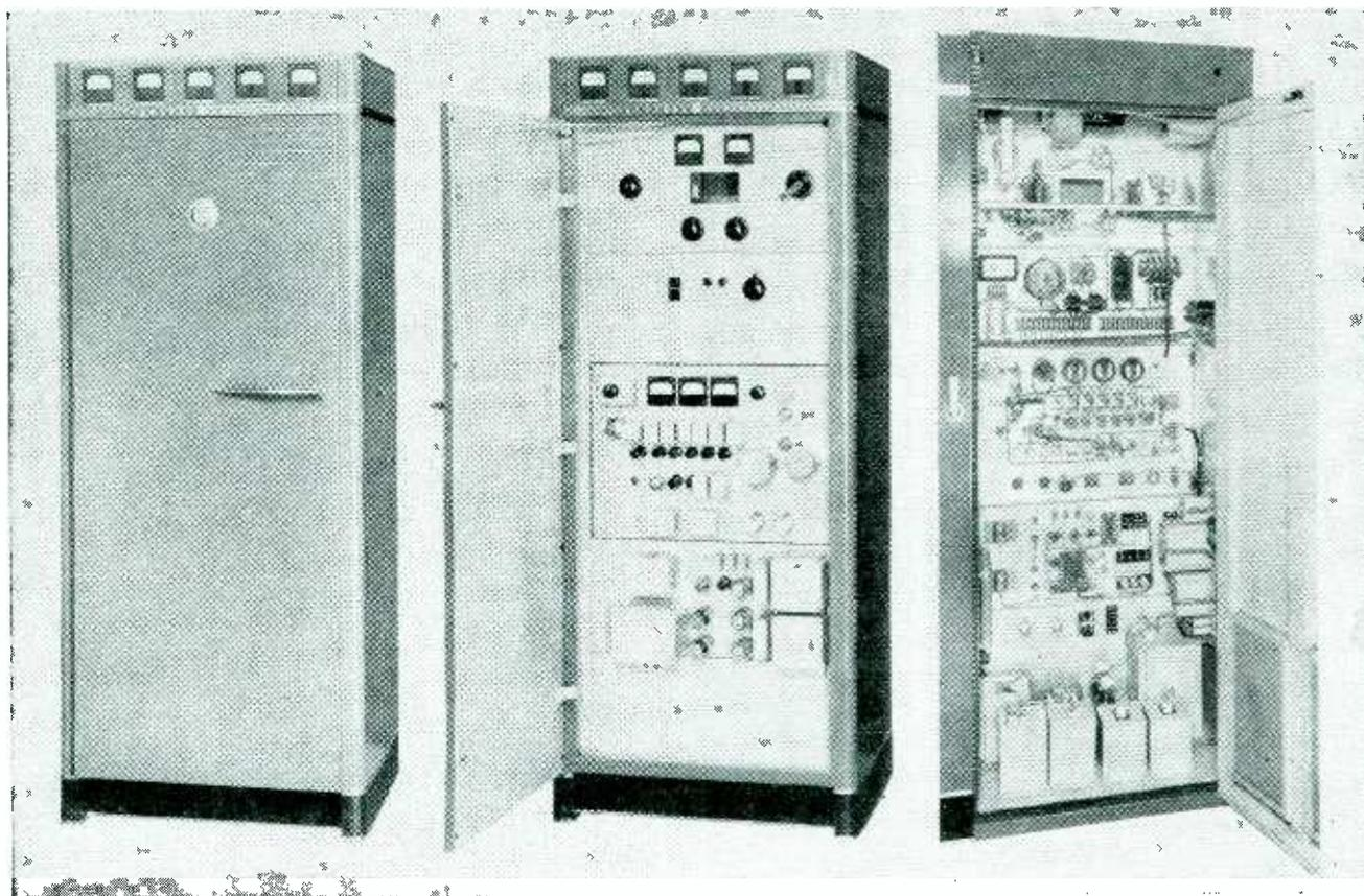
Front and rear views of the complete 250-watt f-m broadcast transmitter. Two power supplies are mounted in the lower section of the cabinet. Overload, time-delay, and high-voltage-shorting relays protect equipment and personnel
