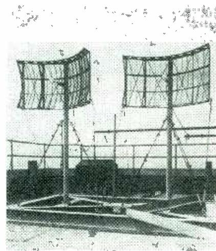
Transmitting and receiving antennas of the Raytheon microwave relay system atop the Lincoln Building, New York City
