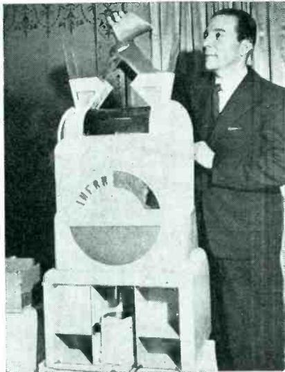
Automatic roasting of coffee completely and uniformly is done in less than two minutes with radiant energy by the machine shown with its inventor, August S. Torres of Medellin, Columbia. Electronic elements of the unit are shown after covers are removed
