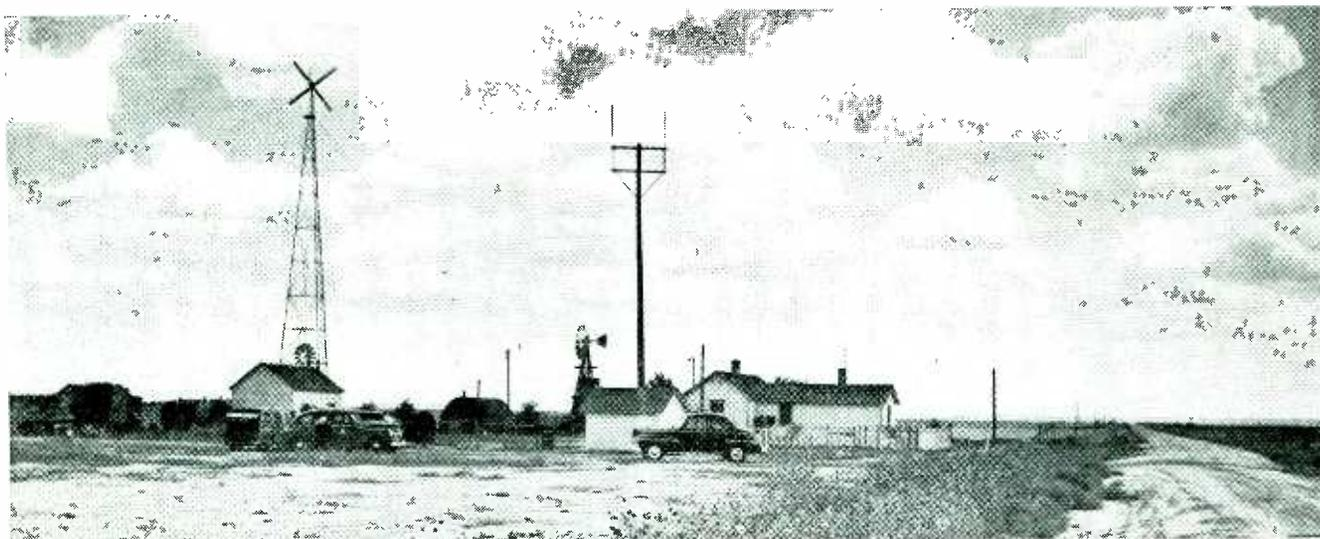
Two-pronged pole supports separate sending and receiving antennas of rural radiotelephone equipment installed at ranch of Cecil F. Blackwelder, about 20 miles from Cheyenne Wells, Colorado. Wind generator unit at left supplies electric power for ranch and radio. Seven other ranches in this area have been linked via radio with the nation's telephone system by Mountain States Telephone and Telegraph Co. (See p. 270 of July 1946 ELECTRONICS for further details)
