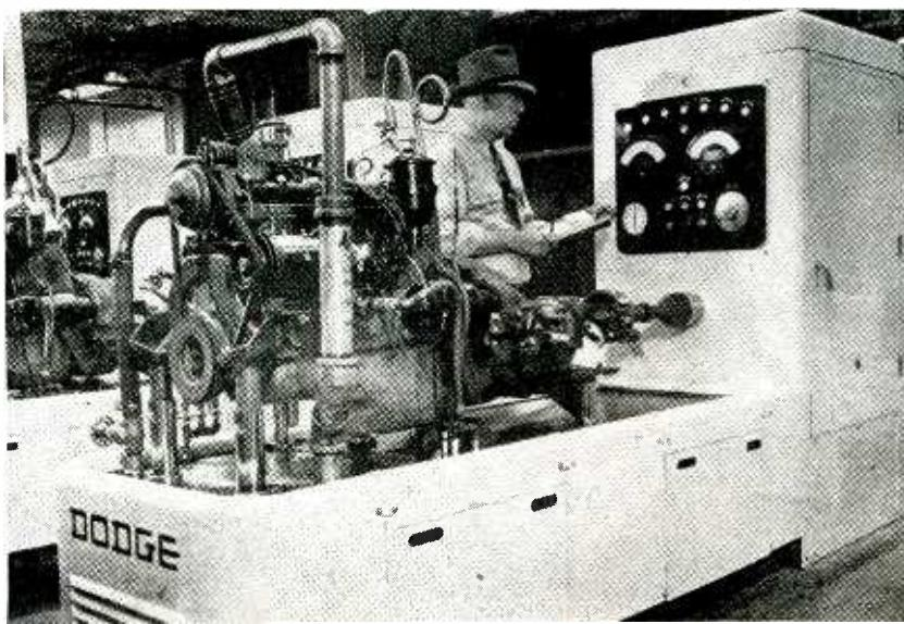
Dynamic testing of Dodge automobile engines is being accomplished by sixty electronically controlled test stands. Above, an inspector checks meters showing rpm, horsepower developed, and 14 other indicators
