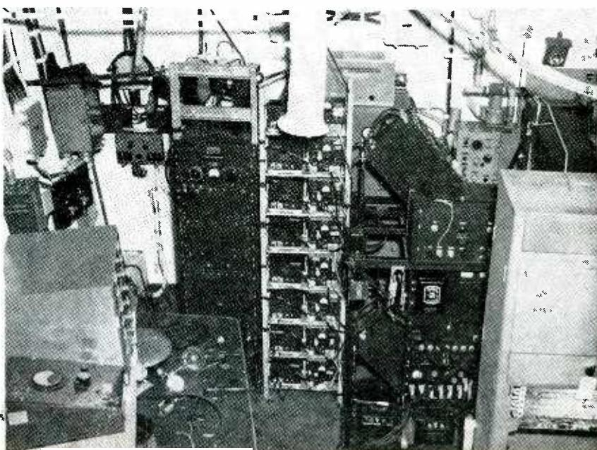
THE PURPOSE of the electronic program of Operation Crossroads was twofold: (1) to expose electronic equipment of the Navy and the Army to the effects of atomic bombs and to assess the damage, and (2) to provide electronic systems for measuring and observing the technical effects associated with bomb explosions, such as water and air pressures, radio wave propagation, wave heights and the like.
