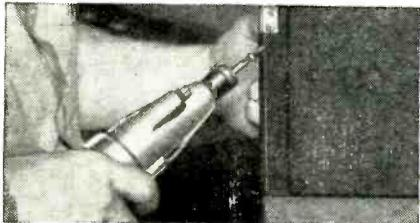
**"One-Hand Driving Is Easy With the Phillips 'Engineered Fit'.** The precision recess snugs right onto the bit of the power driver and sticks there, making it so easy for the operator to center the screw in the hole that he can hold the work with one hand and drive with the other.
