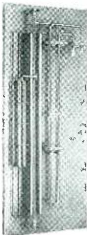
initial f-m antenna installations are often faced with the problem of feeding the new antenna without short-circuiting the a-m radiator or
