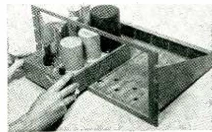
when the amplifier unit is locked into place by one or two levers. A family of amplifiers used in various broadcast station functions is available in the proper dimensions for the new mounting. Six preamplifier chassis units, for instance, fit on a single shelf.
