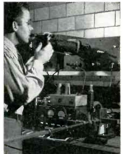
FIG. 2—Photographing microwave absorption bands as displayed on cathode-ray tube
