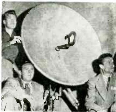
Waveguide and reflector of RCA microwave radio relay transmitter, set up near ring of Mexico City's 60,000-seat bullring for beaming first televised bullfights to a hotel six miles away
