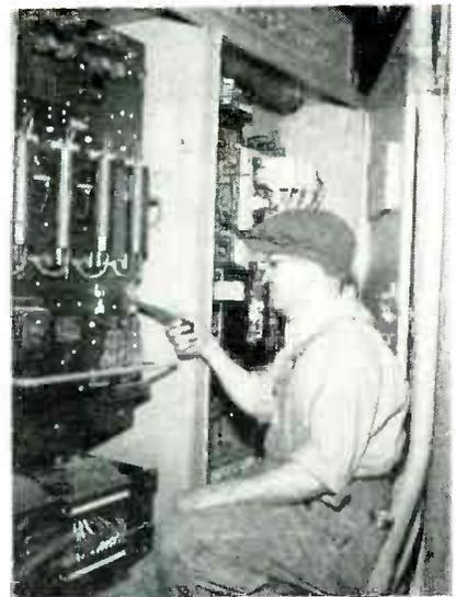
FIG. 7—Complete control equipment for crankshaft grinder. Vacuum-tube section occupies left-hand bay
