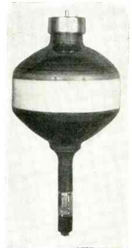
The modified cathode-ray tube has a long-persistence phosphor on a cylindrical screen. When mounted in a strong perpendicular magnetic field and slowly rotated, the tube displays a continuous pattern of the speech wave
