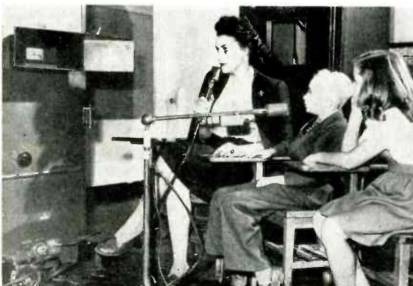
Professor Harriet Green speaks into the microphone. Patterns of the speech waves move across the screen of the special revolving cathode-ray tube, the screen of which is at the left inside the light shield. Joyce Arnold and Richard Hudson read the patterns
