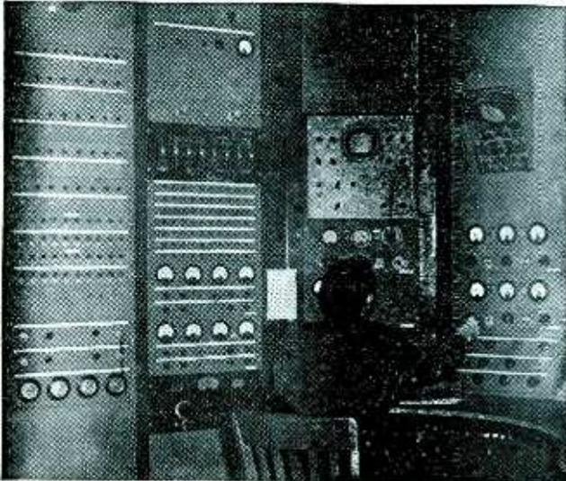
At main control position are vacuum gages, interlock lights, vacuum-pump flow sheet, shortwave receiver for monitoring oscillator, and oscilloscopes showing oscillator frequency and dee potential against time
