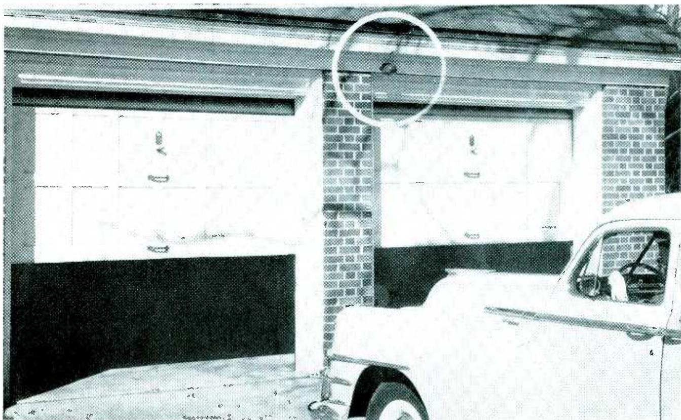
Typical installation of microphone on two-car garage, between doors (in circle). Driver pushes button on dashboard after turning into driveway, and doors are open by the time the car reaches them if approach is made at normal slow speed
