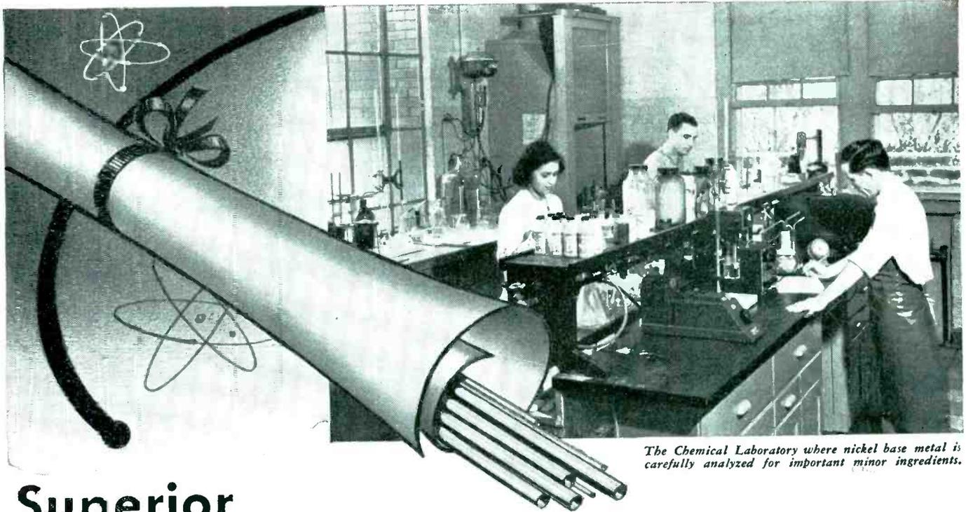
*The Chemical Laboratory where nickel base metal is carefully analyzed for important minor ingredients.*
