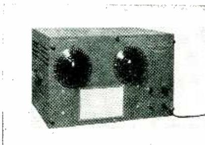
brated every megacycle can be obtained using a new generator with an attenuator adjustable from 20 to 134 db below 1 volt. A calibrated dial drives a piston attenuator. Gears are chosen such that the dial calibrations are 1 db apart. Changes in attenuation have negligible effect upon frequency and vice versa.
