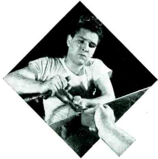
**CHERRY BLIND RIVETS** reduce pounding hours to fleeting minutes. There's no hammering or bucking because they are installed with a **controlled pull from one side of the work only.**
