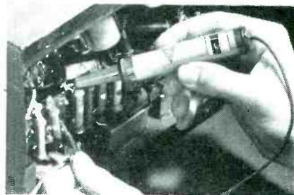
a new ohmmeter that is direct reading between 0 and 10,000 ohms. The equipment illustrated uses a small Weston meter and a standard pen-light dry cell.
