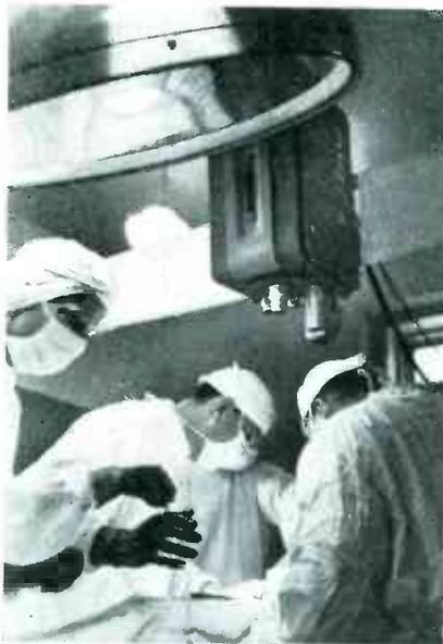
The three-lens television camera, requiring no special lighting, is installed on a track above the operating table. The microphone mounted just behind the camera picks up the running commentary of the operating surgeon. RCA equipment was used
