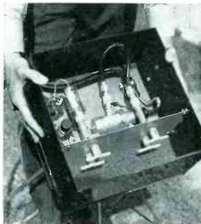
Close-up view of the electronic portion of the speed cop for clocking motorists (ELECTRONICS, July 1947, p. 148). The transmitter is at right with its antenna; the receiver is at left. An insulating panel protects the antennas from damage
