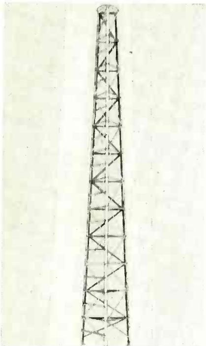
61ST aluminum alloy. Delivered knockeddown, it can be erected by one man. It is designed for low cost developments in the f-m, a-m, and television broadcast fields.
