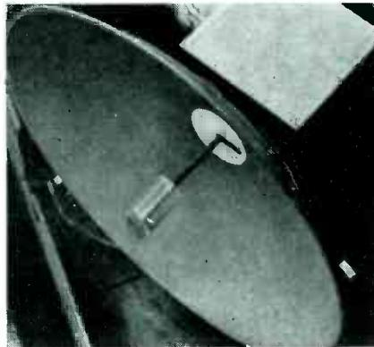
New York microwave relay transmitter (in the box) and beam antenna. Each relay receiver and transmitter is similar in appearance
