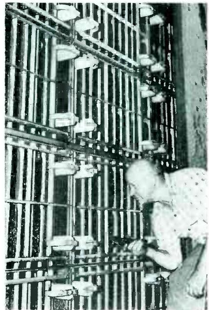
FIG. 1—Airborne particles receive a positive charge as they pass through this ionizer unit
