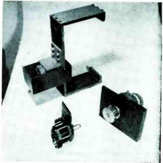
Sinewave p-m generator at lower left, ten-horsepower hydraulic motor at right, and induction generator for tachometer feedback at top
