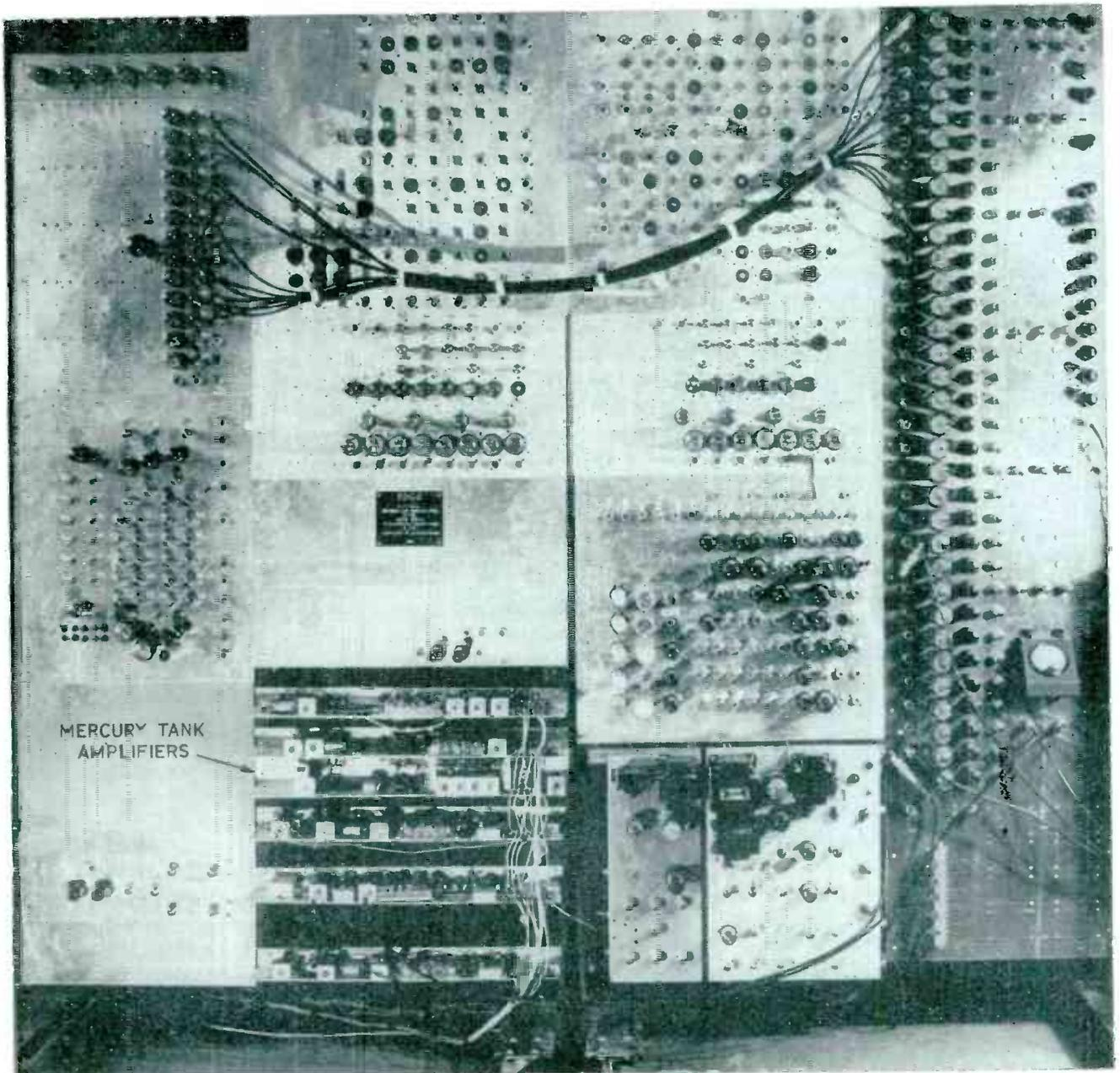
Mercury delay lines are installed in heavy thermal-conducting holders behind this pilot model of the 3,000-tube EDVAC automatic computer. The final model will use mercury lines in glass tubing about 2-ft long, providing 384 microseconds delay
