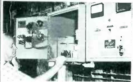
FIG. 3—High-voltage power supply for the precipitator units
