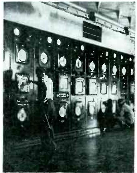
Scores of electronic, pyrometric, and pneumatic instruments are mounted on the four walls of this air-pressurized control room to direct 500 control points in the giant new catalytic refining unit built by Gulf at Philadelphia
