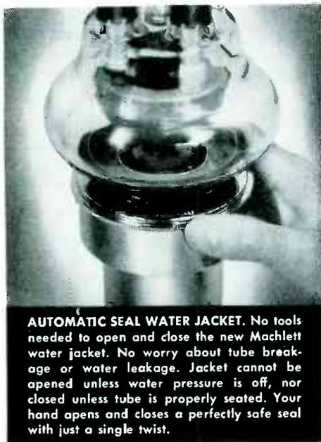
**AUTOMATIC SEAL WATER JACKET.** No tools needed to open and close the new Machlett water jacket. No worry about tube breakage or water leakage. Jacket cannot be opened unless water pressure is off, nor closed unless tube is properly seated. Your hand opens and closes a perfectly safe seal with just a single twist.
