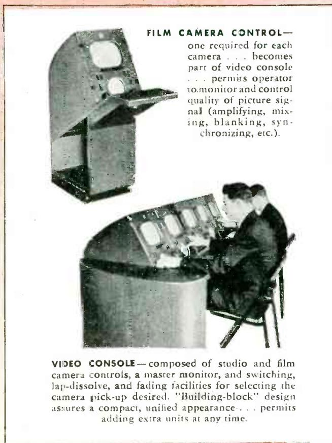
IT IS NOW POSSIBLE to use two film projectors . . . and a slide projector with just *one* film camera . . . and to switch instantly from one to another *without moving the camera*.
