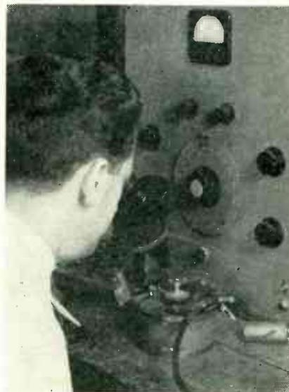
FIG. 3—Sources of microphonics are detected by vibrating tube and observing motion of internal parts
