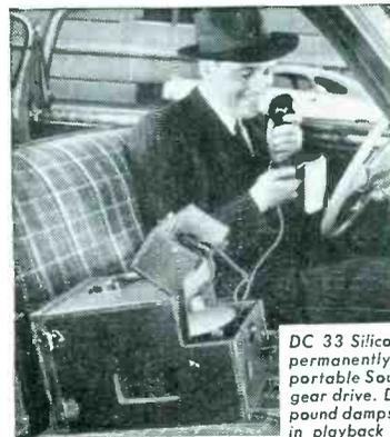
DC 33 Silicone Grease permanently lubricates portable SoundScriber gear drive. DC 4 Compound damps vibrations in playback head.
