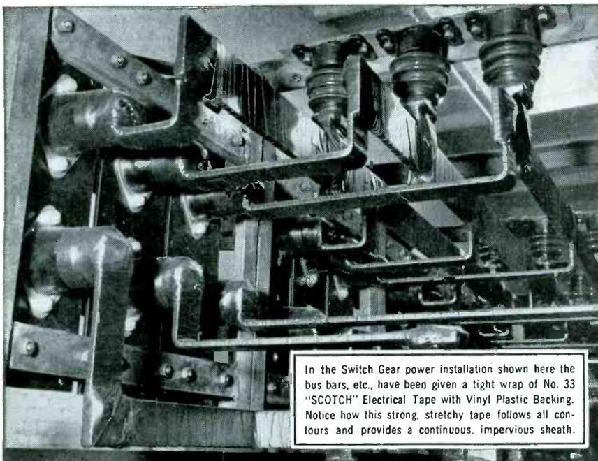
In the Switch Gear power installation shown here the bus bars, etc., have been given a tight wrap of No. 33 "SCOTCH" Electrical Tape with Vinyl Plastic Backing. Notice how this strong, stretchy tape follows all contours and provides a continuous, impervious sheath.
