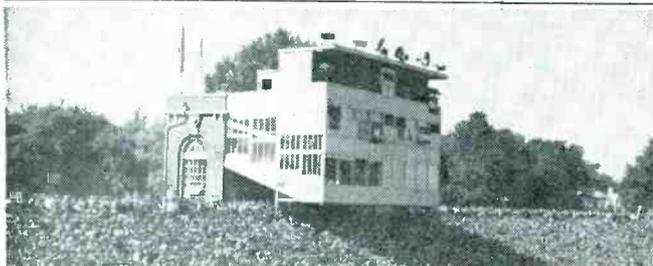
University of Michigan stadium, Ann Arbor, Mich. Altec Lansing large multicell horns driven by Altec Lansing 1/4 KW amplifier, are centralized over press stand, override noise level of 86,000 spectators. Reiss Public Address Systems, Detroit, contractors.
