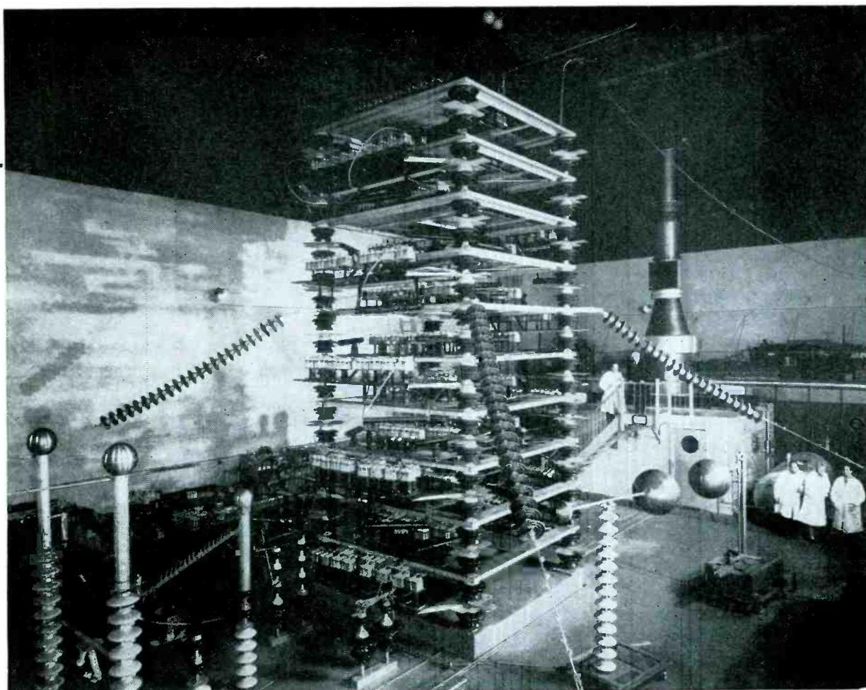
Experimental capacatron used in the tests
