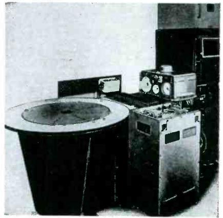
FIG. 2—Large-screen plan position indicator used by British Admiralty
