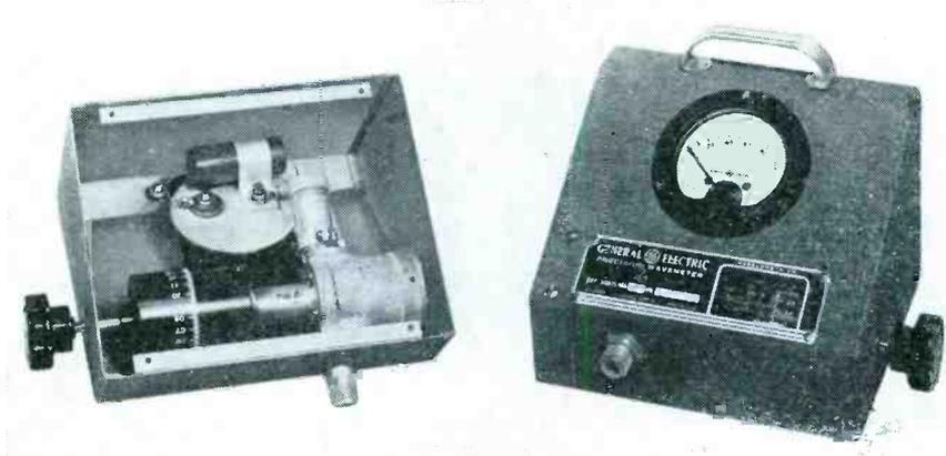
Postwar re-entrant line short-circuit type of wavemeter for use in the frequency range from 8 to 12 cm, as described below
