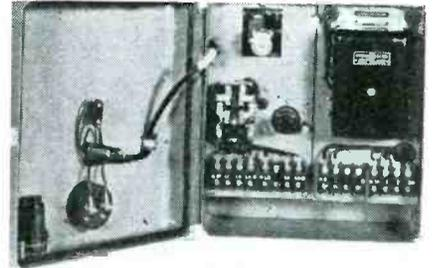
combustion control system for commercial oil burners comprises master, phototube, and electrode units. The system shuts off fuel flow immediately if oil fails to ignite or if the flame is extinguished after successful ignition. Write for bulletin GEA 4779.
