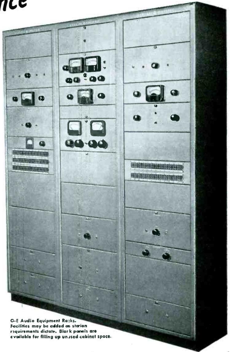
G-E Audio Equipment Racks. Facilities may be added as station requirements dictate. Blank panels are available for filling up unused cabinet space.
