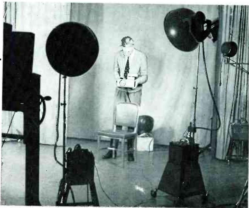
Light meter is held at position to be taken by subject and is aimed at flash lamp, which is tripped remotely by pushbutton on end of cord
