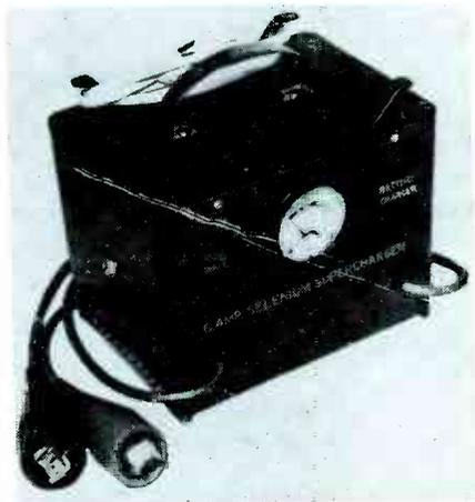
portable battery chargers. Each unit features a direct-reading meter, circuit-breaker protection and selenium rectification. They operate on 110 volts, 50 to 70 cycle a-c current.
