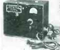
78E Standard Signal Generator, 50 to 7 Mc. Unmodulated or with 400 cycle modulation.
