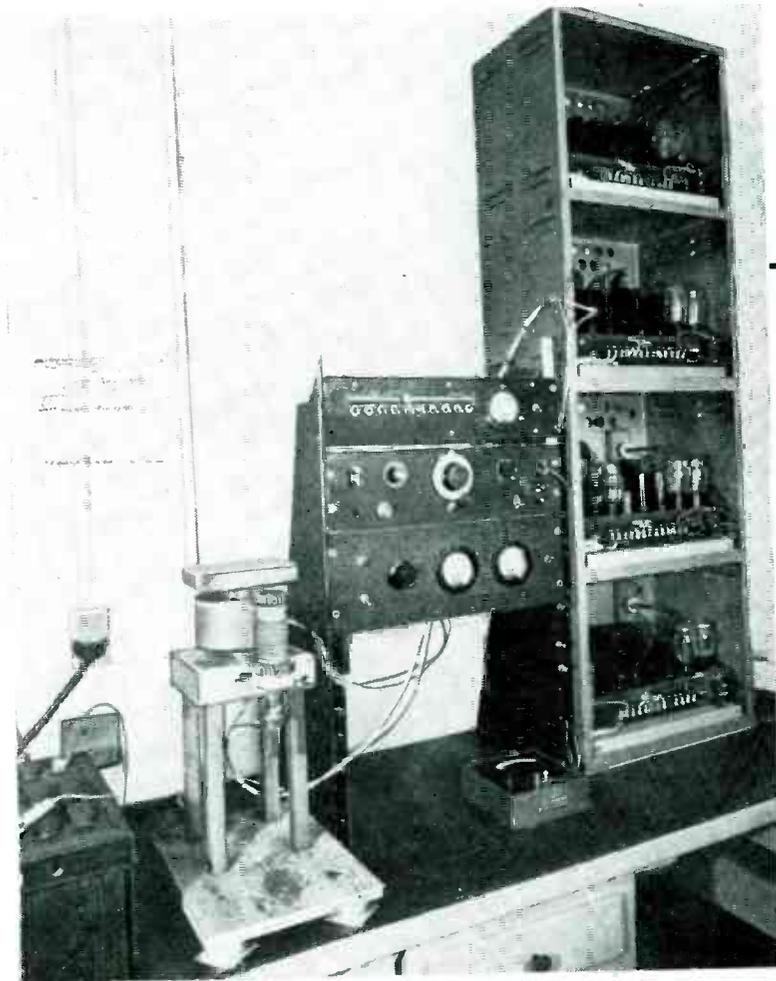
FIG. 1—Experimental sonodizing setup. Left to right: 24-volt polarizing battery; magnetostriction transducer and soldering iron; unit containing oscillator, loading capacitors, and controls; four 50-watt amplifiers
