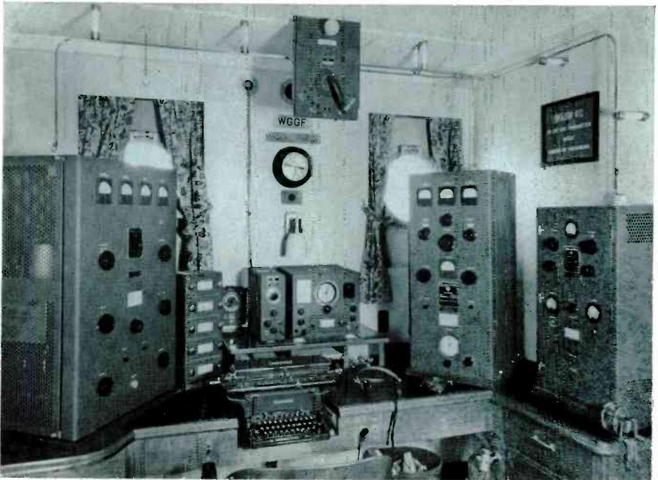
Typical shipboard installation of distributed type. Shown from left to right are the main transmitter, coil rack, emergency crystal receiver, intermediate and high-frequency receiver, high-frequency transmitter, and emergency transmitter
