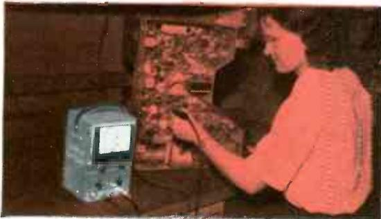
THE RCA WV-75A HIGH-FREQUENCY VOLT OHM YST employs a push-pull dc vacuum-tube voltmeter circuit that provides excellent linearity and stability. It will measure dc resistances up to 1000 megohms, ac and dc voltages up to 1000 volts. A newly developed diode probe and internal circuit permits readings of both positive and negative peak voltages at frequencies up to 250 Mc.
