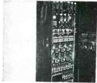
Elevator-control thyatrons and resistance-capacitance circuits are in the lower portion of the rack that houses the rectifiers (top) for the signaling system
