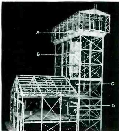
Housing for accelerator accommodates 150-ton crane (A) to lift pressurized generator (B) so that vital parts can be adjusted, stack of annular steel plates and insulators (C) inside which beam is formed and accelerated toward deflecting magnet (D) that directs beam into target room (E) where nuclear reactions will be produced
