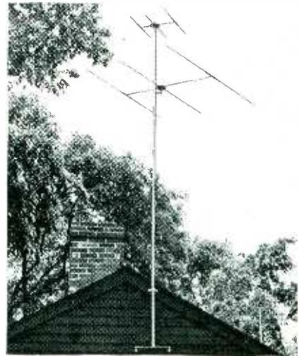
on a single mast and designed for reception of all channels operating in a particular area. Elements are constructed of half-inch aluminum tubing. More arrays can be added to the installation as additional stations go on the air.
