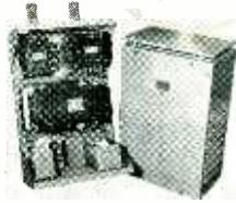
Mfg. Raytheon; Navy CR1-201407; Pri: 92-138 v., 15 amps; Sec: 65 cy., 1 phase. Sec: 115 v., 7.15 amp., .82 KVA, .96 PF. Contains the following components:
