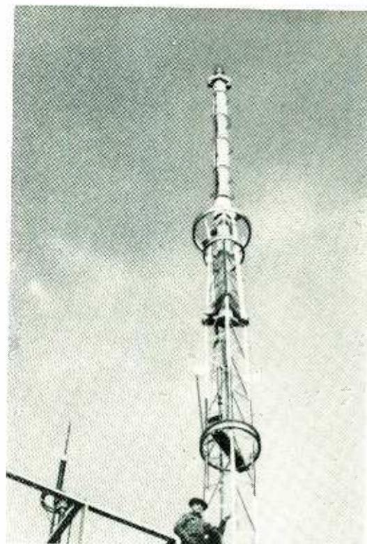
Circularly polarized antenna in use by radio station WHKX
