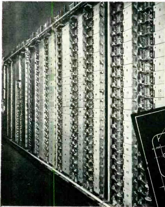
Selector Switch Frames—a part of the 15,000—line installation of Federal Rotary Telephone Switching Equipment at the Rochester Telephone Corporation, Rochester, N. Y.
