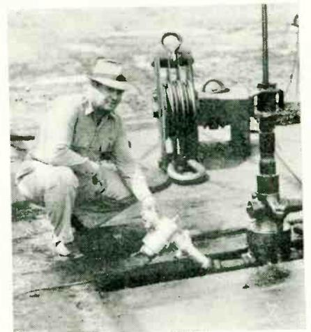
Well attachment ready for firing. Sound traveling down is partially reflected by obstructions and surface of oil
