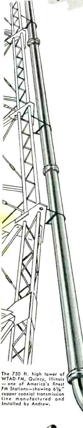
WTAD-FM did. That's why they selected Andrew  $6\frac{1}{8}$ " coaxial transmission line. In spite of the 800 ft. long run, including a 750 ft. run up the tower, *the overall efficiency is 90%!*
