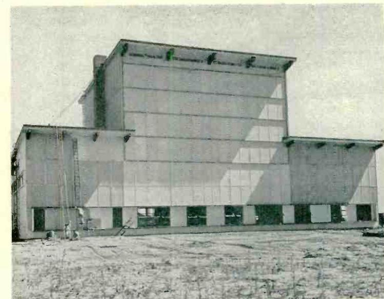
**ROOM FOR RADAR**—Nonmetallic structure nearing completion at back of Park, for testing huge radar antenna arrays regardless of outdoor weather conditions. Even sprinkler system inside is removable for sensitive tests
