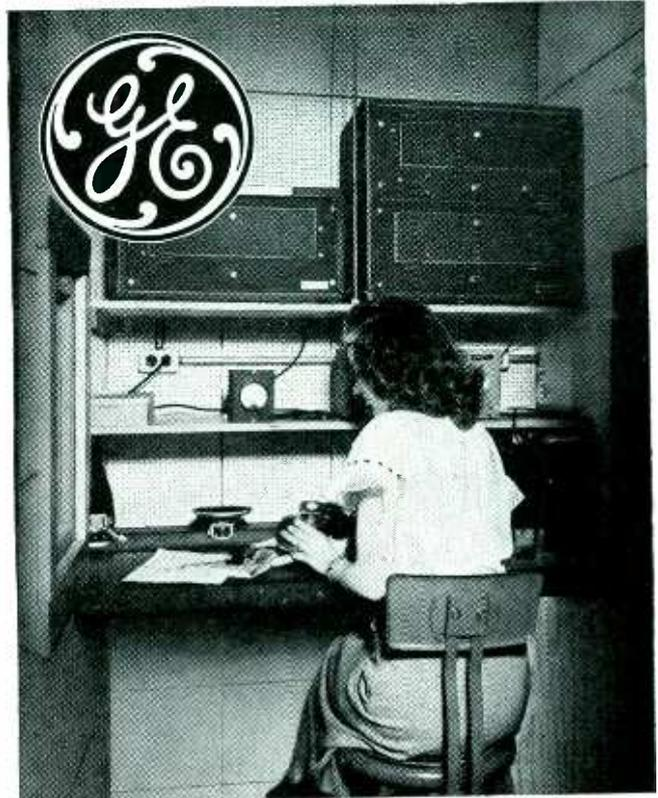
Finished speaker test for buzz, spurious response and acoustical characteristics.
