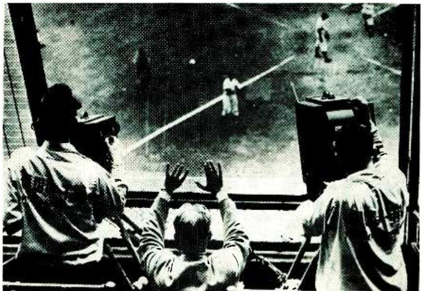
This 7 x 8-ft slab of Plexiglas was recently installed by the Cadillac Plastic Co. of Detroit at Briggs Stadium in that city as a protection for television equipment. The ½-inch sheet will offset the impact of a 9-ounce ball travelling at over 100 miles per hour, according to researchers at Rohm & Haas Co., Philadelphia, makers of Plexiglas
