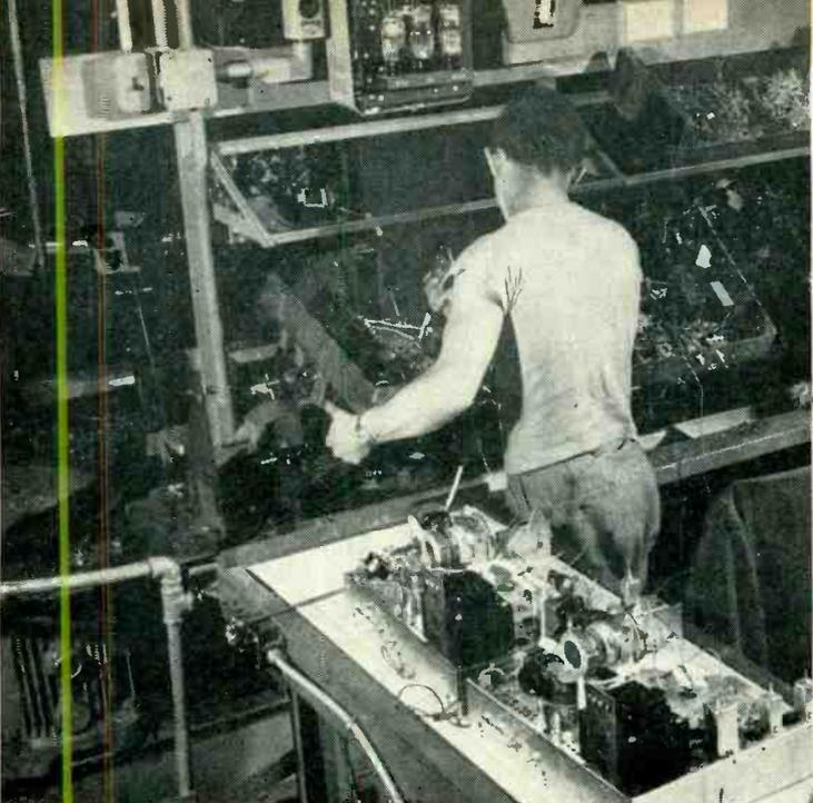
**ELECTRONICS DOES IT**—Thyratron-tube control for drive motor of endless conveyor on television line (above head of man, with cover removed). Speed control knob is alongside. Crossover conveyor in foreground brings sets from end of first line (off picture at lower right) to start of second line
