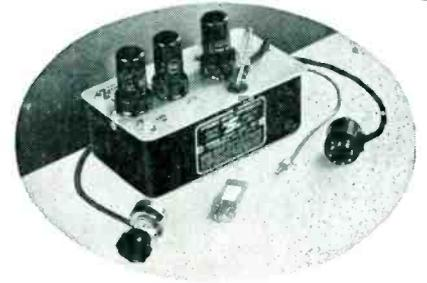
The remote control, for setting the exact degree of suppression you find most pleasing, can be mounted wherever you wish . . . at the instrument or even in another part of the room. The 3-tube suppressor unit can be placed anywhere in the cabinet.
