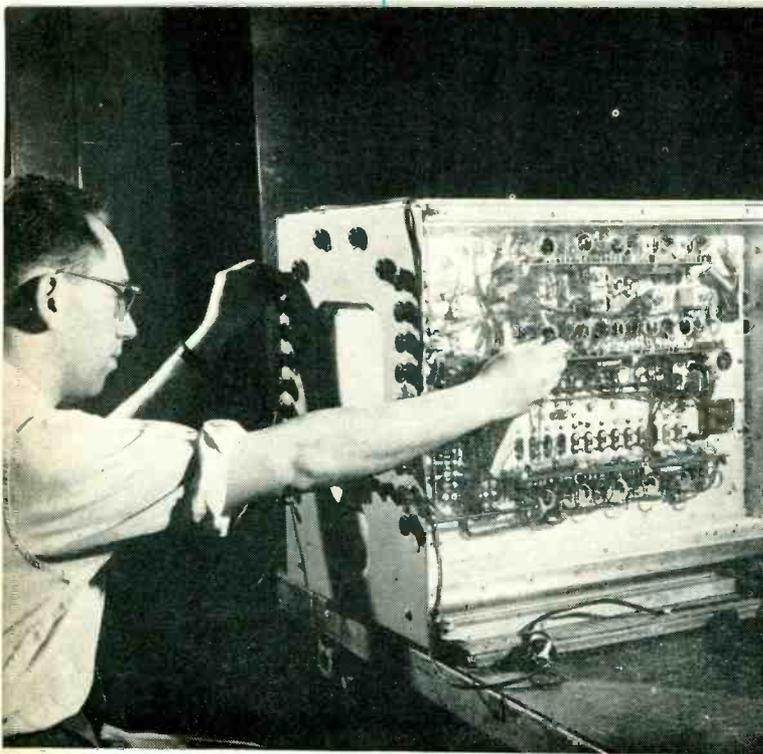
**MEASURING THROUGH LUCITE**—Test program engineer checking television monitor unit by inserting prods through holes over dangerous high-voltage terminals. Transmitter test section has now been in operation over a year without an accident
