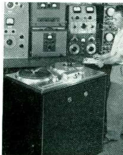
signed expressly for f-m broadcast service, the new Ampex tape recorder has a response within plus or minus 1 db between 30 and 15,000 cycles as well as other features designed for broadcast facility. Tape speed is 30 inches per second and the unit has a time capacity of 35 minutes.
