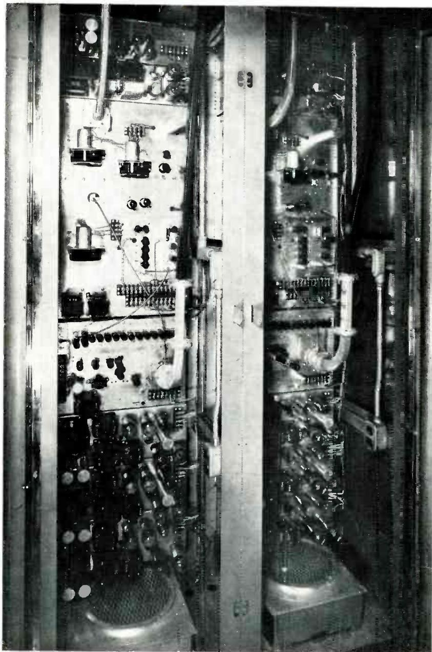
Rear view of a pair of 6,000-mc repeater racks at Neshanic
