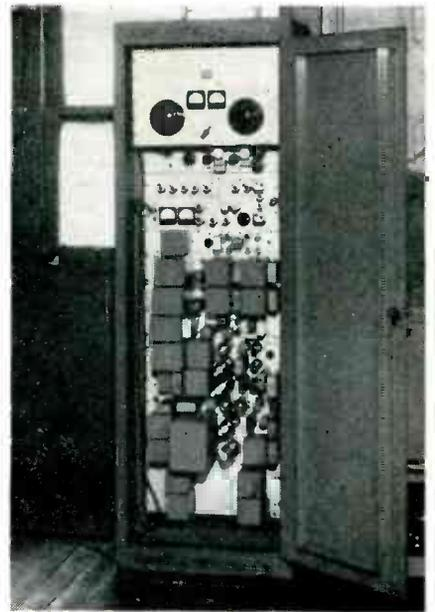
Sperry transmitter and receiver and power supplies used at both ends of the beam installation
