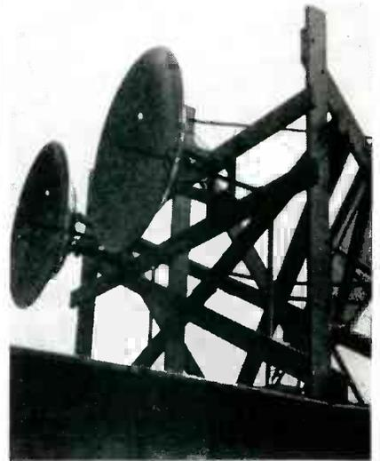
Four-foot parabolas installed on the roof of Jamaica station for beam transmission and reception
