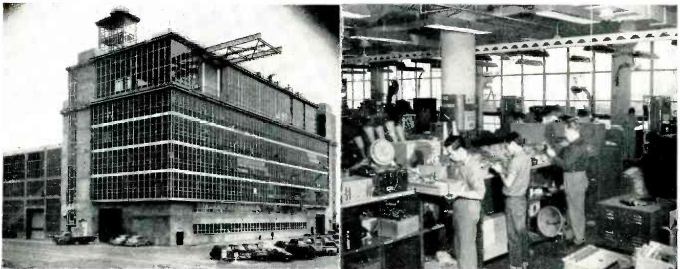
Nearly two acres of exterior glass provide daylight illumination for civilian technicians in the Navy's new six-story Ordnance-Electronics and Optical Building, San Francisco. Building contains an escalator extending from main to third floors, and a 39-foot outrigger crane capable of a 15-ton lift from railroad track at ground level. In the radio and repair section (right), all marine communications equipment is overhauled and tested
