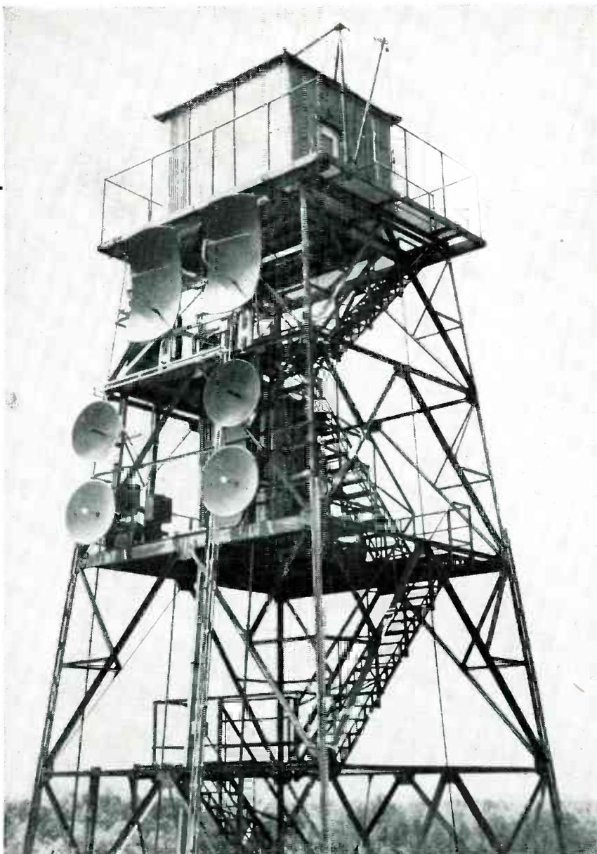
Antennas, horns, and waveguides installed on Western Union tower at Neshanic, N. J.
