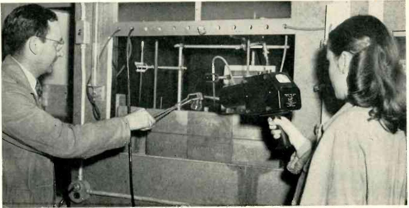
Use of radiation survey meter for monitoring hot samples during preparation of radioisotopes for industrial uses. This provides a continuous check of the efficiency of techniques and materials used to protect personnel against excessive radiation exposure
