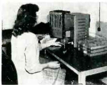
the potency of antibiotic by electronic means. Since the potency is proportional to the diameter of the area inhibited by the antibiotic in a germ culture, the diameter is measured by recording elapsed time between selected interruptions of a light beam scanning the inhibited area under study while the area is moving at a constant known speed.
