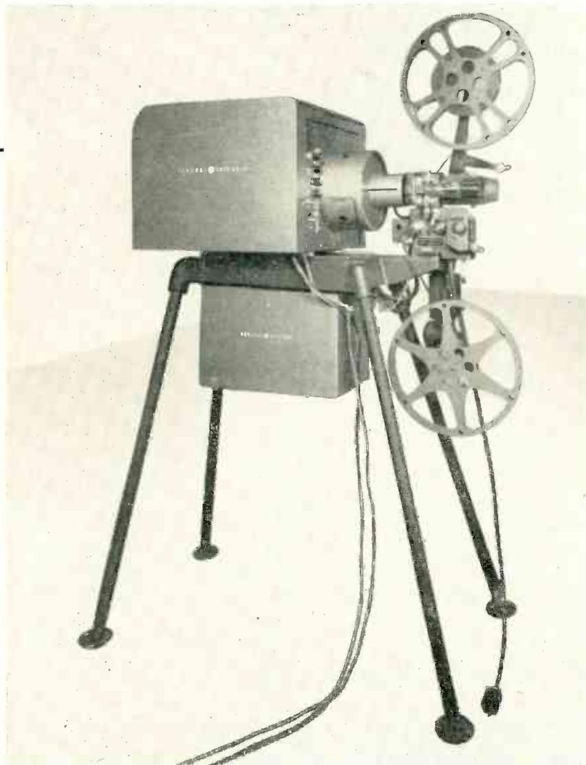
Complete television film projector. The speed-control amplifier is mounted in the suspended cabinet
