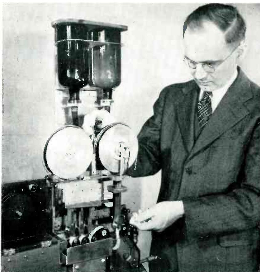
Charles Kunz of Kodak feeds a leader strip through the experimental high-speed hot developing machine used at the receiver
