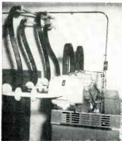
Top of cabinet installation at Neshanic, showing complete antenna switch for 6,000-mc television relay system
