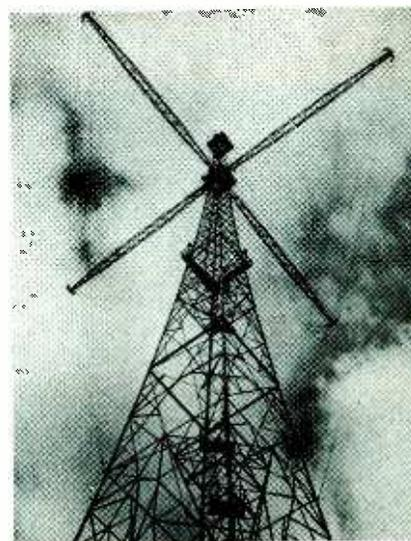
A view of the 325-ft steel lattice transmitting tower at the master station of the Lane Identification system, Puckeridge, Herts., England. Transmissions go out automatically at one-minute intervals 24 hours a day, seven days a week, so ocean-going ships approaching Britain can fix their position and set their receivers for the subsequent voyage up channel
