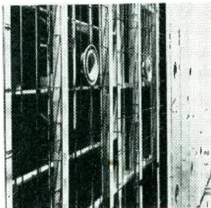
Adjustable combination supply and return air diffusers serving main floor of manufacturing building at Western Electric's Allentown plant
