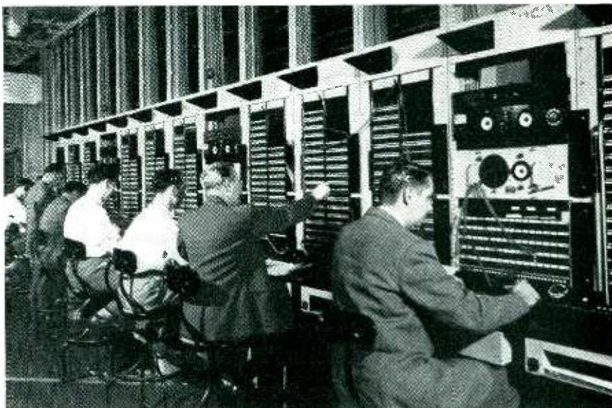
Long-lines technicians monitor the workings of the new electronic equipment for dialing long-distance calls
