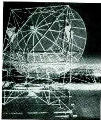
Giant parabolic reflector above KTSL, atop 1,600-ft Mt. Lee, Calif. Television shows originating in Hollywood studios, whose lights are seen in the background, are beamed directly to the 16-ft saucer, which has a focal length of four feet
