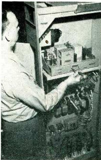
FIG. 5—A Wilcox vhf transmitter is adjusted after overhaul in the test rack
