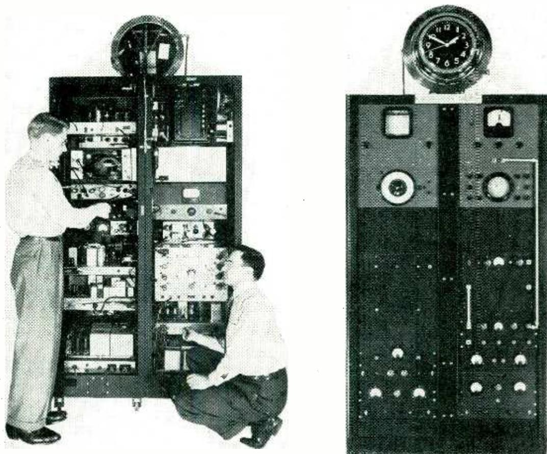
Rear (left) and front (right) views of the Bureau of Standards clock. The tubing containing ammonia gas is wound in a helix around the large clock at the top
