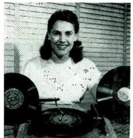
Two pickup arms and a speed-adjustable motor permit this record player to handle conventional records, as well as those of Columbia and RCA Victor. The large diameter hole of the latter is accommodated by a brass collar that slips over the normal spindle. Developed by Scott Radio Laboratories, Inc. of Chicago, the player is automatic on 78-rpm disks and manual on long-playing types
