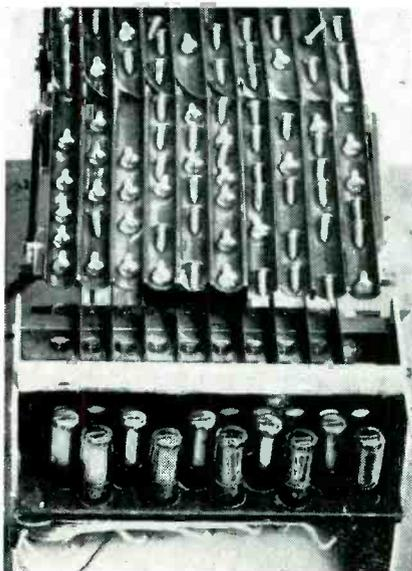
Ten paralleled phototubes view separate holes through which screws fall at rates as high as 6,000 per minute. Circuit resolves and totalizes simultaneous counts
