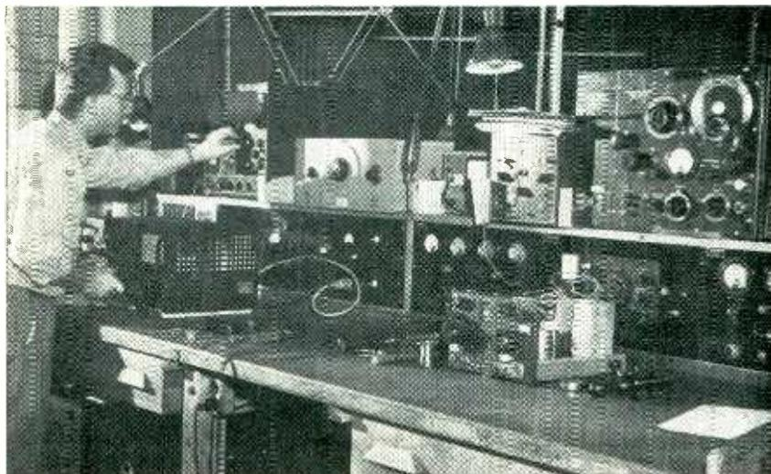
FIG. 9—Receivers employed in overseas flights are tested with this equipment
