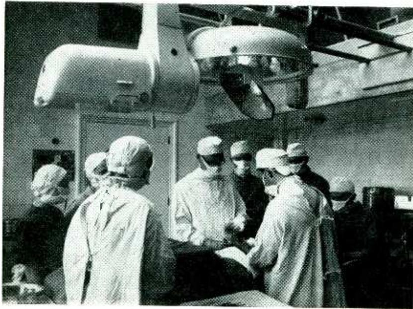
General view of the operating theatre in Guy's Hospital, London, shows the unobtrusive character of the television camera installation (upper left). The camera is attached to the lamp over the operating table and both are moved on an overhead track
