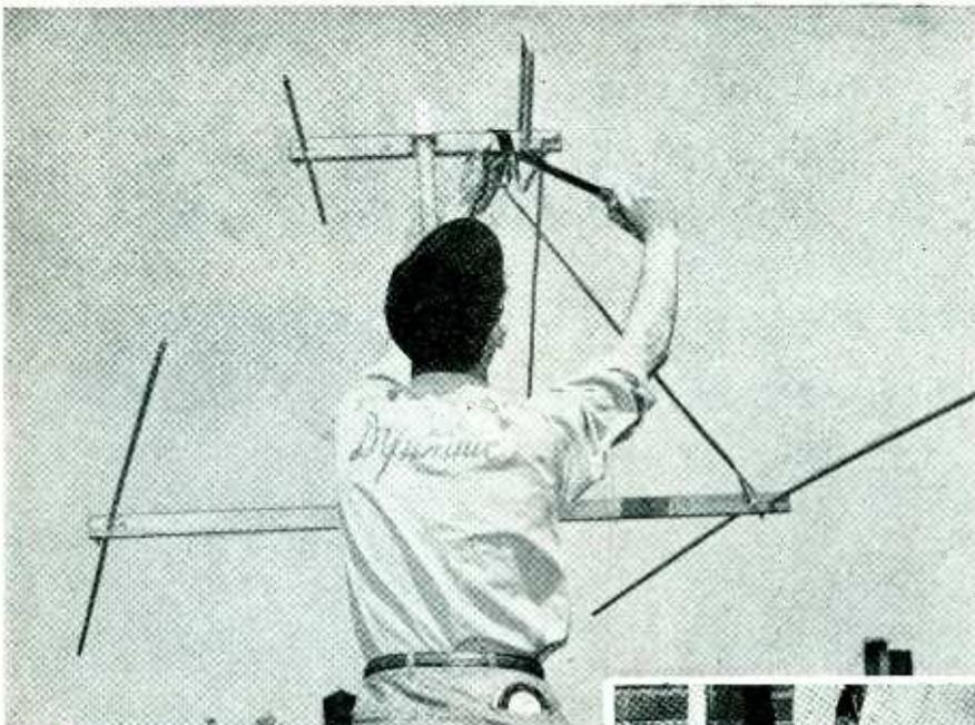
**TAPING LEAD-IN CABLE** to TV antenna cross-beam with plastic-backed No. 33 "SCOTCH" Electrical Tape. Easy-to-apply tape helps prevent "snow" streaks on receiver screen by insulating and fastening cable securely.
