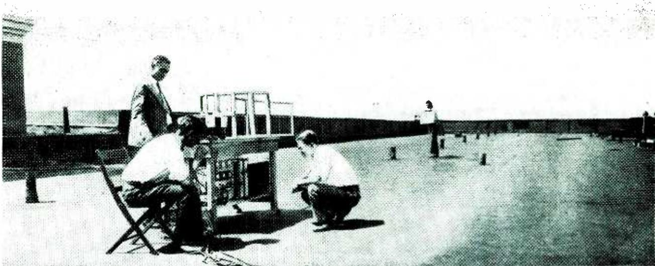
Taken in 1928, this picture shows a laboratory test of the FH-11 oscillating magnetron being used as a voice-modulated microwave transmitter at 400 mc. The art was not ready for such a development, and many years had to pass before a radio
