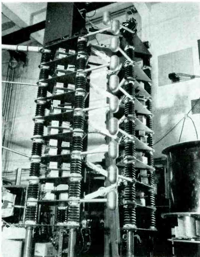
An 8 stage capacitor-rectifier multiplier. This unit is used in the "Racetrack" Synchrontron of the University of Michigan
