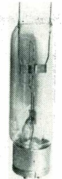
This GE type FH-11 split-anode magnetron was available commercially in 1930 but nobody wanted it
