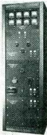
sists essentially of a beam supply, reflector supply, control supply and filament supply. The first three units, delivering d-c power, are well regulated; the fourth, delivering a-c power, is not regulated.
