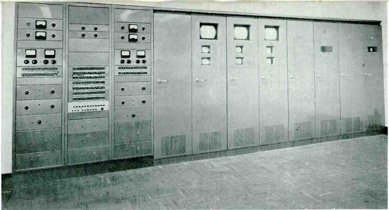
Audio equipment, video monitors, sync generator and associated equipment form the outer wall of the shielded room to the transmitter operator's right
