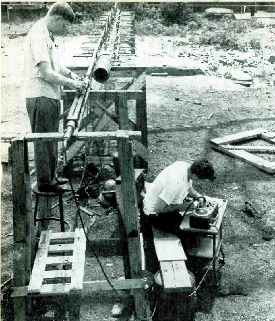
Engineers making final tests of the six-bay superturnstile antenna just prior to hoisting it into place. Man at left reads meter indicating standing waves on slotted-line section. Signal generator on table (right)
