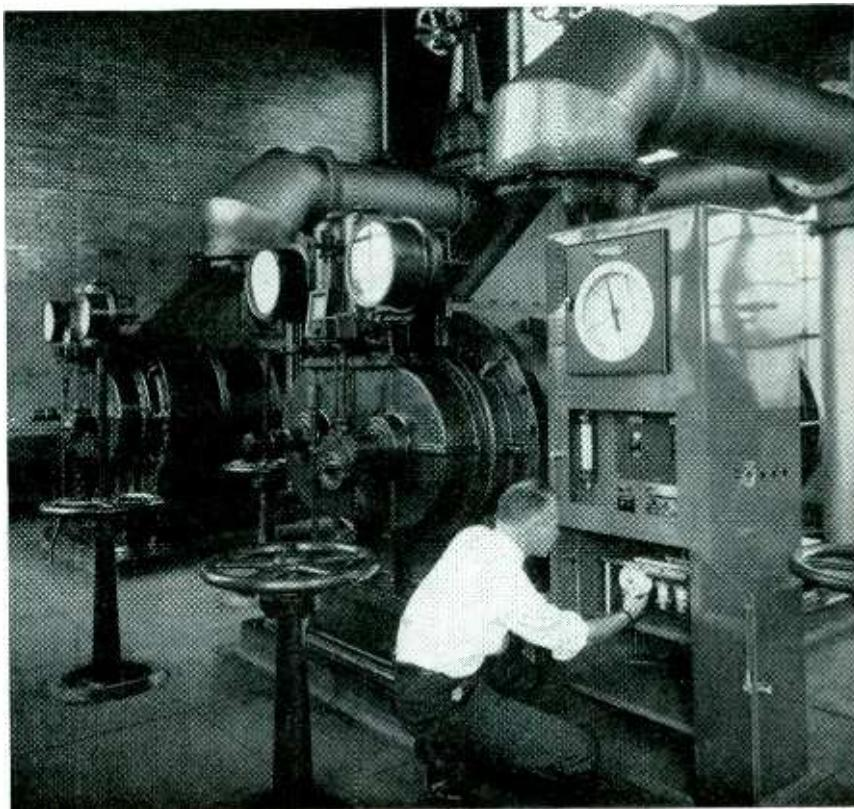
Installation of the analyzer in the metering room of a gas and coke producing company
