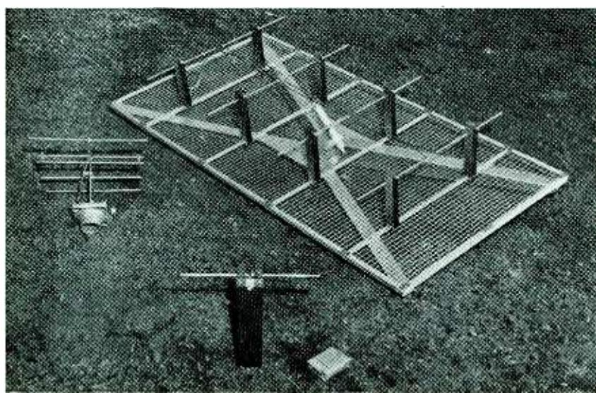
The three types of receiving antennas used in the Washington, D. C. uhf television field strength measurements are shown above. They are the half-wave dipole, a 4-element Yagi and an 8-element array
