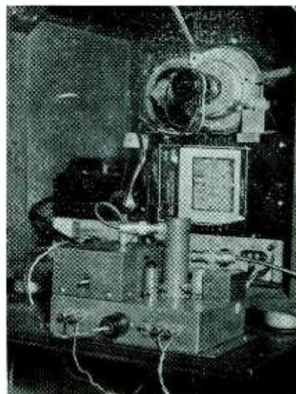
The 500-mc converter used in making the uhf measurements. The coaxial input cavity is mounted next to the oscillator
