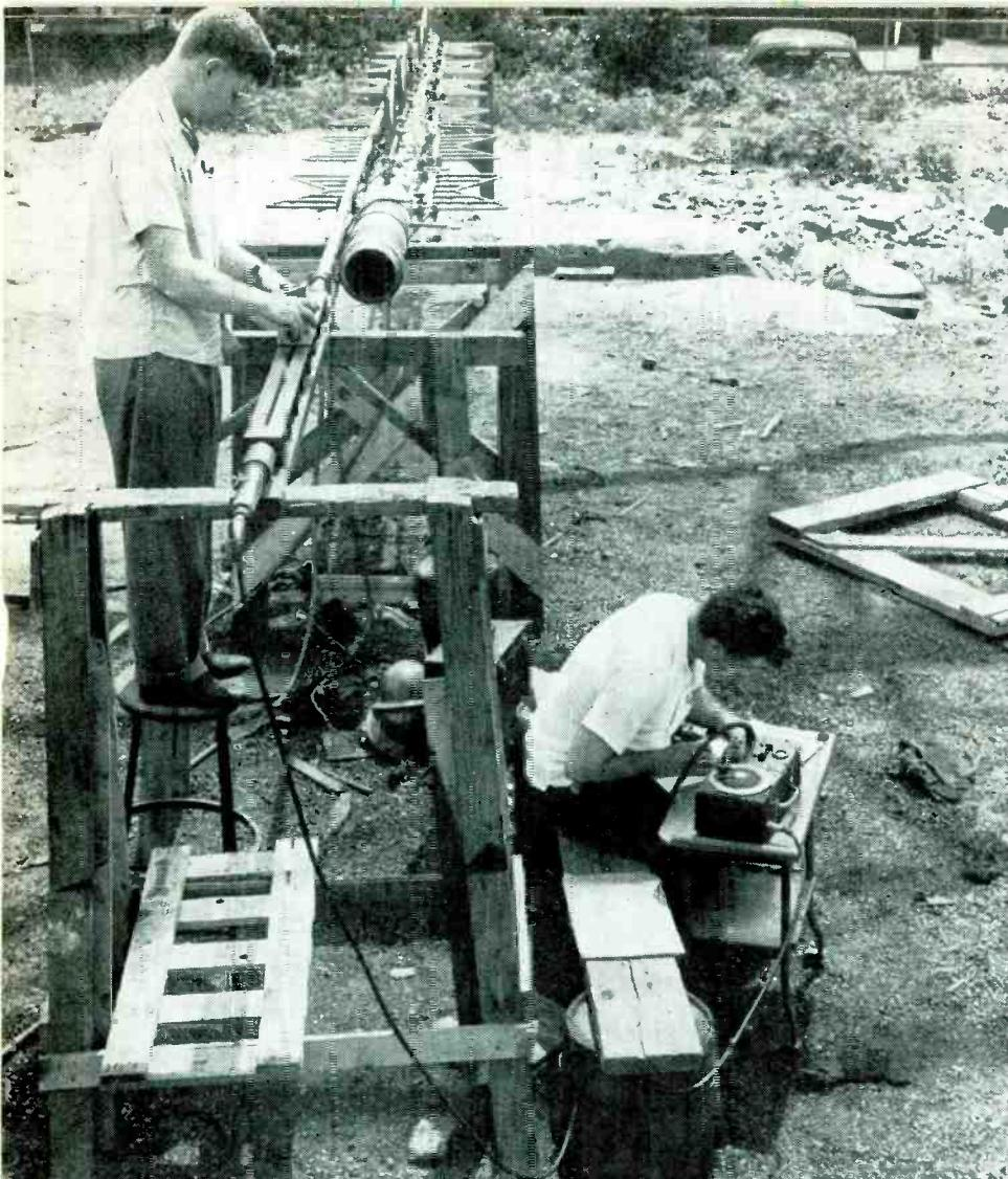
Engineers making final tests of the six-bay supertturnstile antenna just prior to hoisting it into place. Man at left reads meter indicating standing waves on slotted-line section. Signal generator on table (right)
