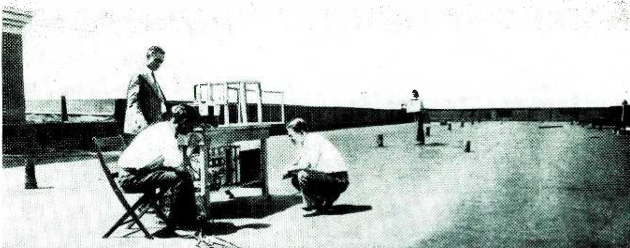
† Taken in 1928, this picture shows a laboratory test of the FH-11 oscillating magnetron being used as a voice-modulated microwave transmitter at 400 mc. The art was not ready for such a development, and many years had to pass before a radio
