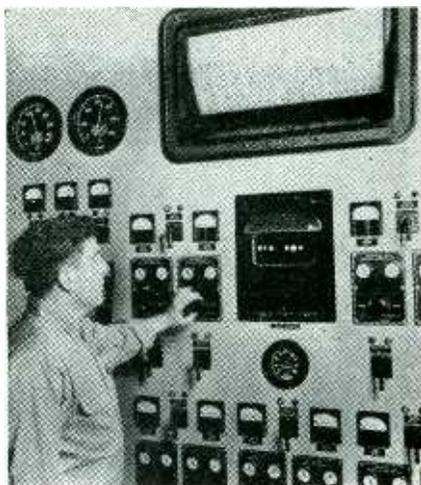
Six glowing discs represent six different flames as viewed by a remotely located camera on the furnace floor
