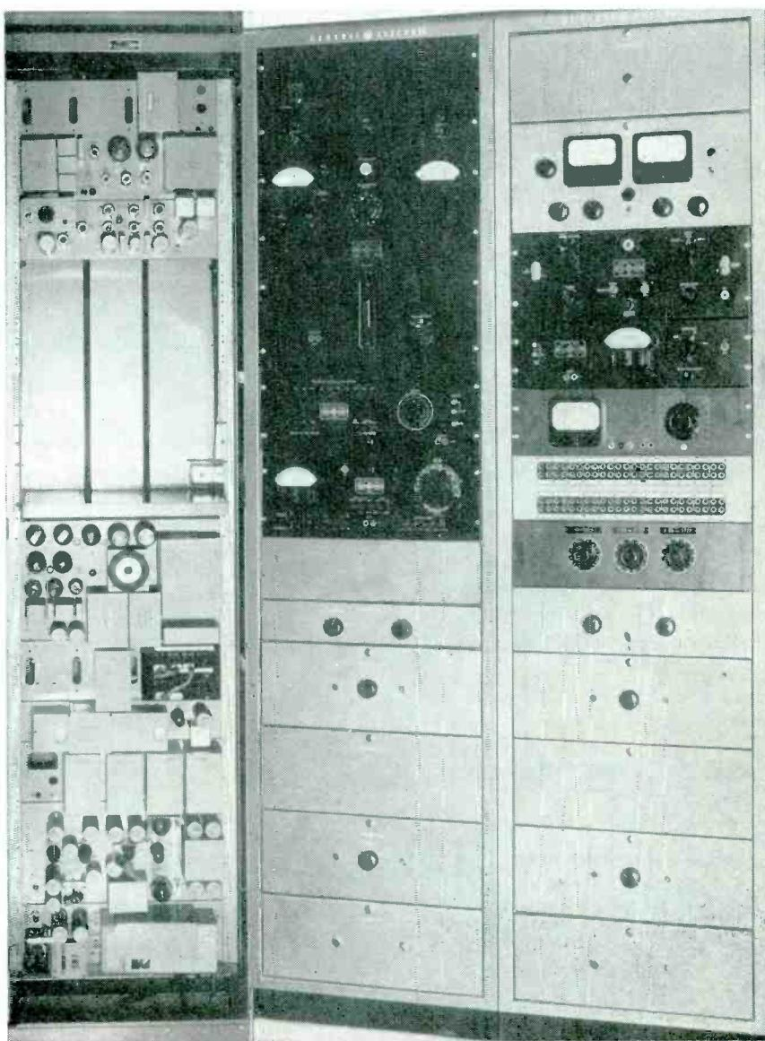
One of the coaxial cable terminal racks (left) and monitoring equipment (right) are located in the hallway outside shielded room
