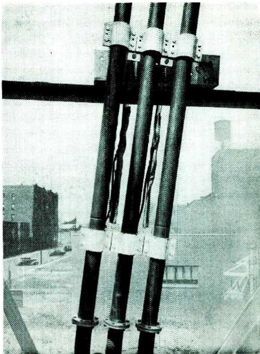
**Coaxial cable hangers compensate different coefficients of expansion of steel tower and copper line. Upper clamps are merely lined with asbestos compound. Lower copper-lined clamps grip coax. Downward thrust is taken by springs. Ground is carried by the copper braid from lower clamp to tower**
