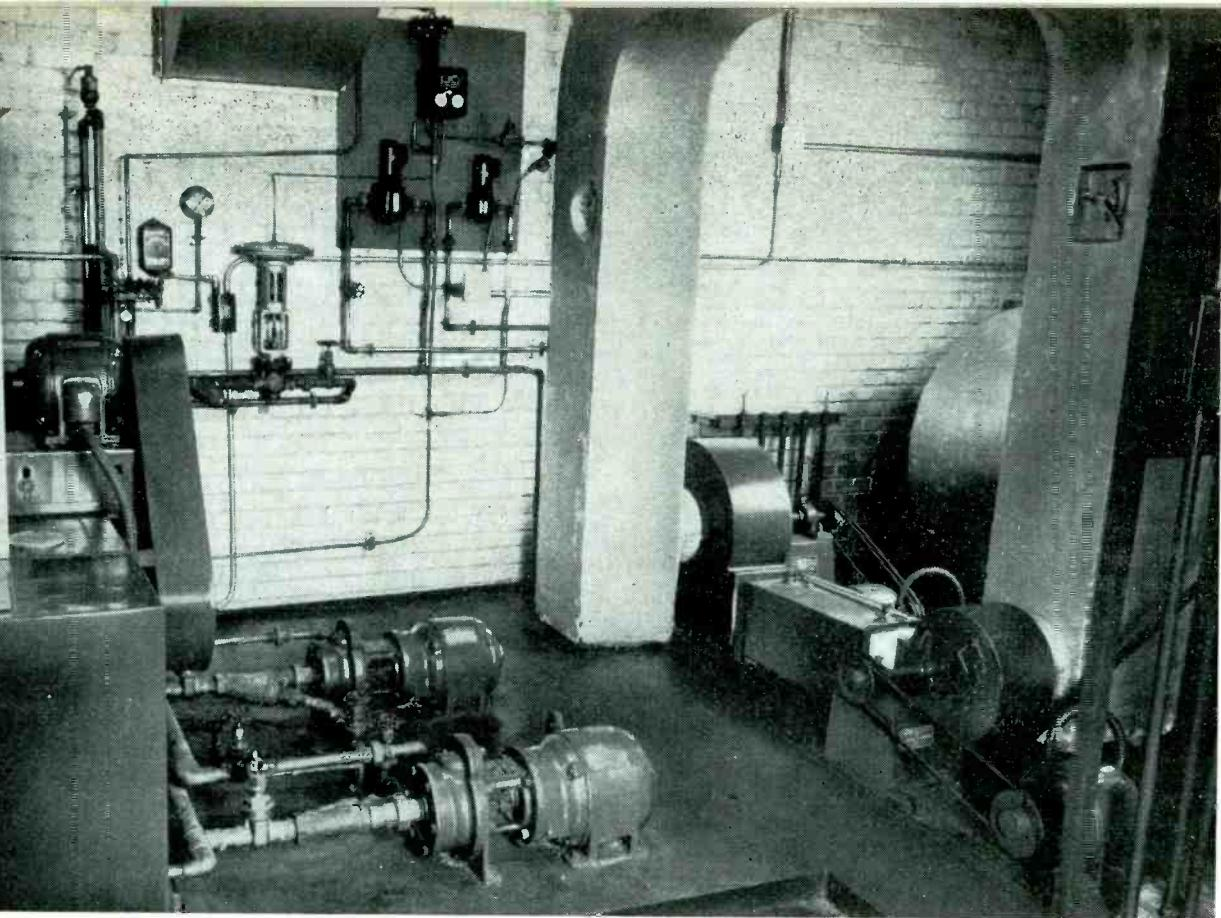
Distilled water cooler, water pumps and cubicle cooling fans in the utility room. Flow control equipment and safety interlocks are mounted on wall at the rear
