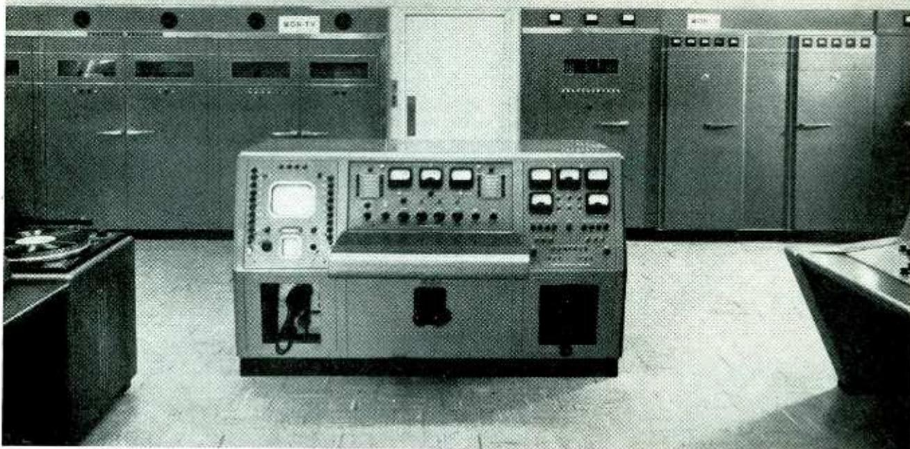
Transmitter control is centered at console in foreground. Television transmitters at left and f-m at right. Turntables and cueing desk just show at left and camera control and mixer desks at right
