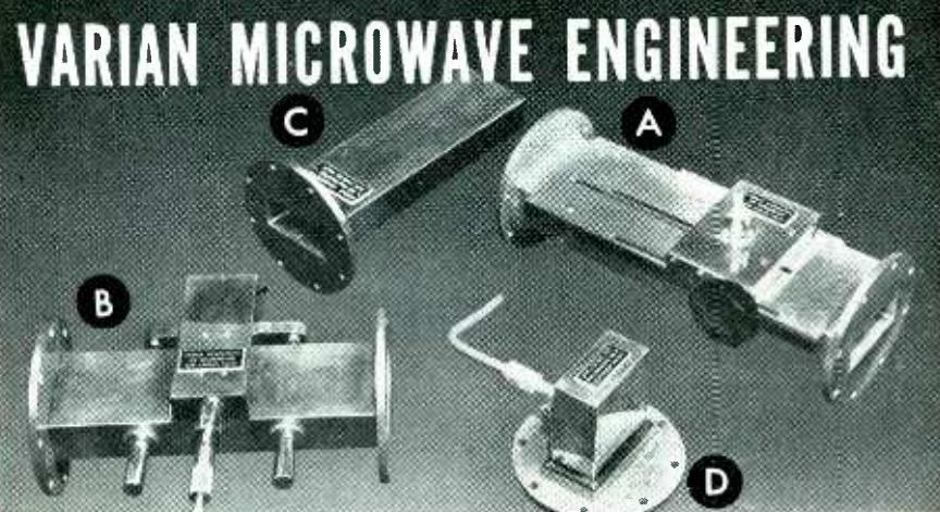
**WAVEGUIDE TEST** equipment for use between 2600 and 3950 mc; 1½ by 3 by 0.080 in.; RG-48/U waveguide with UG-53/U flanges. These and special units for early delivery.
