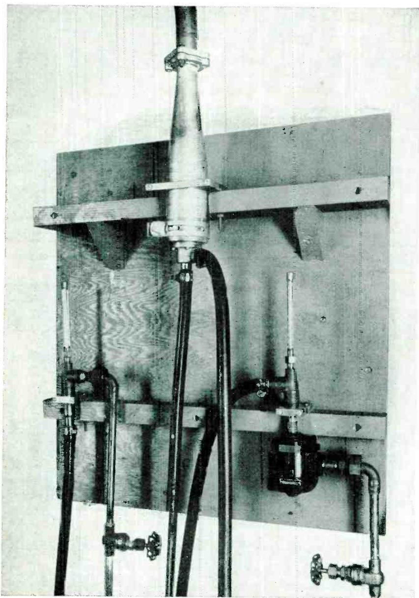
Dummy load used for testing transmitters. Metered water flows over a power-dissipating resistor. Temperature difference of water between input and output shows power
