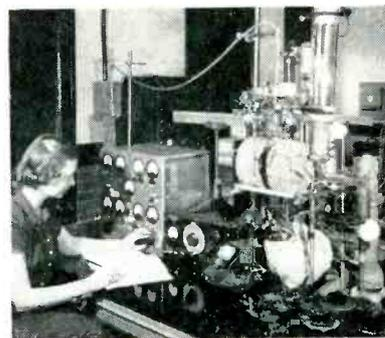
The three-stage nonmagnetic mass spectrometer in experimental operation at the National Bureau of Standards
