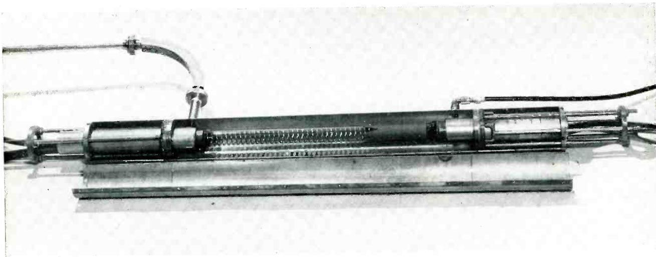
Attenuator at right end of glass envelope suppresses oscillations in 1,000-watt power amplifier
