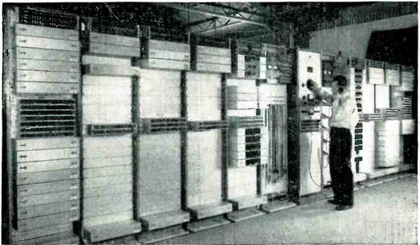
Carrier equipment racks for control station of aeronautical communications network
