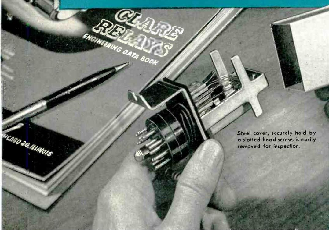
Steel cover, securely held by a slotted-head screw, is easily removed for inspection.
