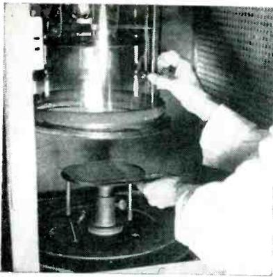
FIG 6—Glass master is placed in sputtering system to form 500-mesh screen
