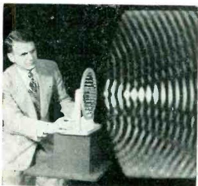
moves through the field, a clear picture of the sound radiation is built up by scanning.
