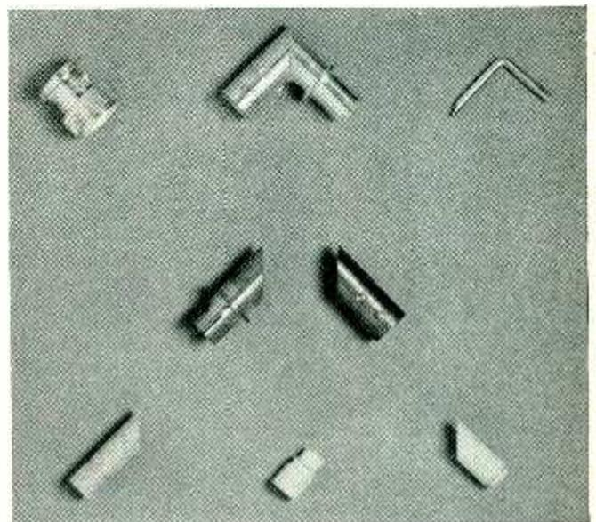
Right-angle connector showing component parts and mitered sections before silver soldering and plating. Teflon dielectric is shown at bottom—Courtesy Industrial Products Company, Danbury, Conn.
