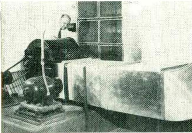
Typical blower and associated ductwork for a broadcast transmitter
