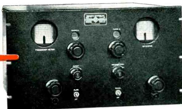
**Type 1108-A Coupling Panel** provides a centralized control panel for quickly and conveniently interconnecting those units of the equipment used in a particular measurement. It carries the necessary switches and volume controls for all operations in making frequency measurements. The bottom panel contains a Type 1105-P1 Speaker for audible monitoring of beat frequencies.
