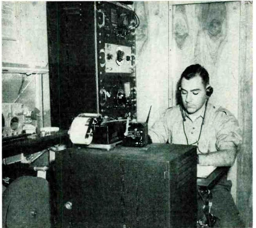
Cosmic-ray radiosonde receiving and recording equipment, inside the trailer
