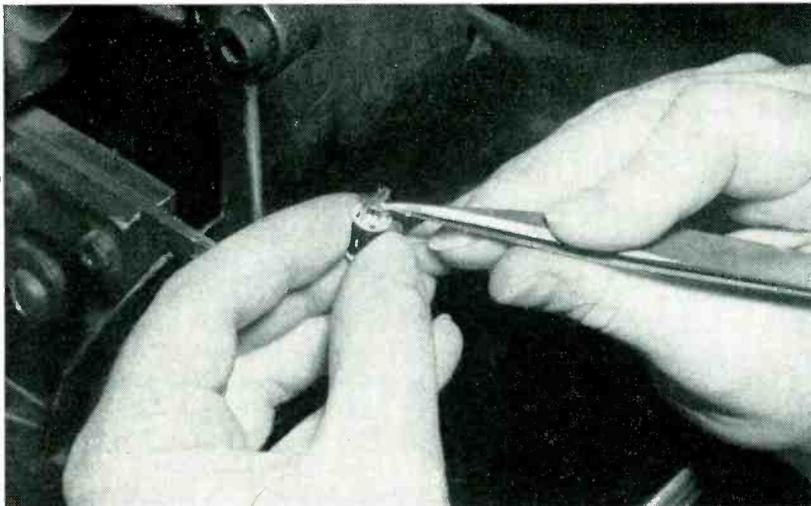
Subminiature tube fabrication requires special skill and over 150 different pieces of equipment. Photograph shows tube mount being assembled at Sylvania's plant
