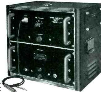
This unit is designed for use as an oscilloscope deflection amplifier for the measurement and viewing of pulses of extremely short duration and rise time, and contains the Video Amplifier Unit, Power Unit and low-capacity probe.
