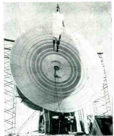
Fifty-foot radio telescope parabola is fabricated from thirty pieces of carefully-machined aluminum
