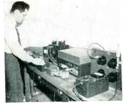
Set-up at National Bureau of Standards for noise figure calibration. At left arm of tee is the noise diode, and the right arm is a two-terminal network simulating the source. At right is a precision attenuator with a voltmeter directly in front of it
