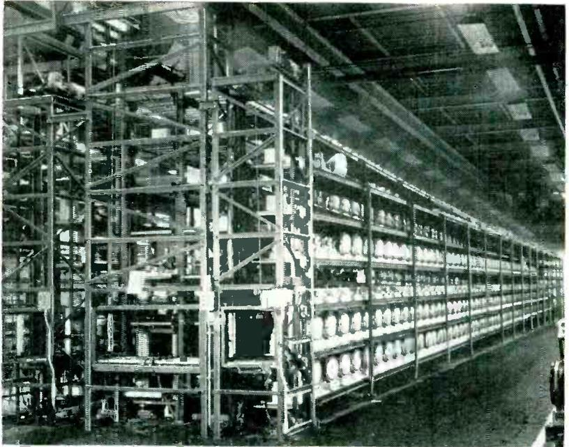
Elevator end of chassis storage conveyor, with all three elevators at the loading and unloading level. Pushing a button brings chassis down automatically from any desired tier
