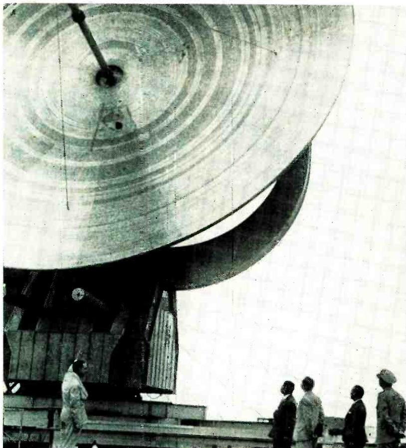
This unusual photograph of the Naval Research Laboratory 600-inch radio telescope was taken on the occasion of a visit by a Japanese legislative, scientific and technical mission. The giant antenna is expected to provide means for studying sun spots and their effect on earth radio and communications
