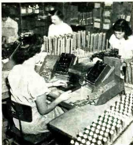
LIMIT BRIDGE FOR TESTING resistance accuracy of Stripohm resistors is operated by Theresa Collura (foreground).
