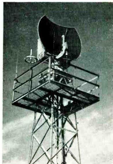
FIG. 3—Airport surveillance radar provides a standby source of video for radar control system
