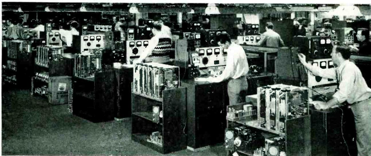
Modern steel desk-type benches replace shielded cages, giving engineering-office atmosphere to test and alignment section of Motorola's production floor. Unit under test fits into recess in surface of bench
