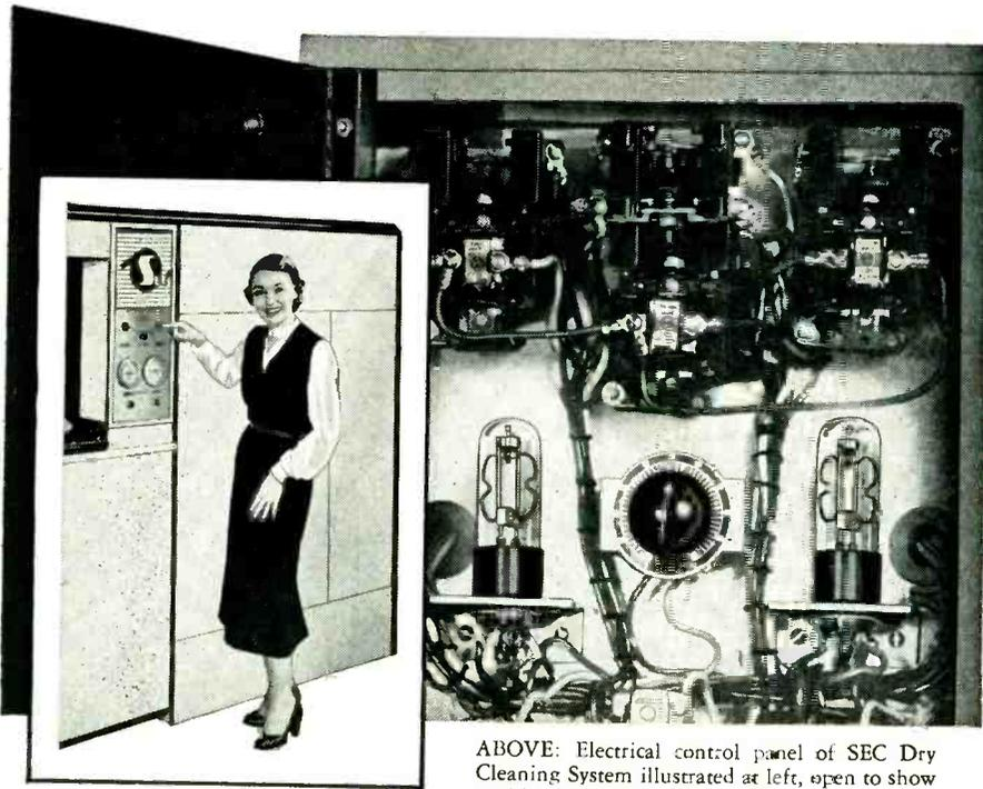
ABOVE: Electrical control panel of SEC Dry Cleaning System illustrated at left, open to show position of EDISON Thermal Relays.
