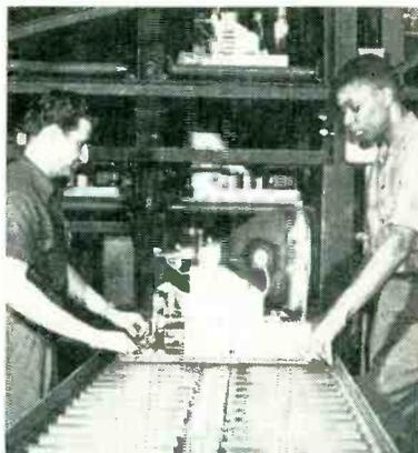
Moving a chassis pan from the portable roller conveyor onto the double-width loading elevator serving the two center tiers of the storage system
