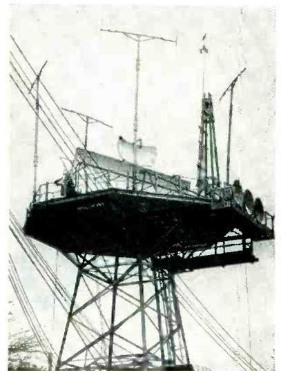
**FIG. 2—Microwave early-warning radar antenna system includes high and low-beam antennas mounted back-to-back**
