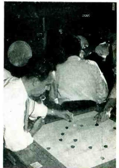
**FIG. 1—Air traffic control center showing aircraft plotted on Skyatron. Two sector-monitoring ppi scopes may be seen in background**
