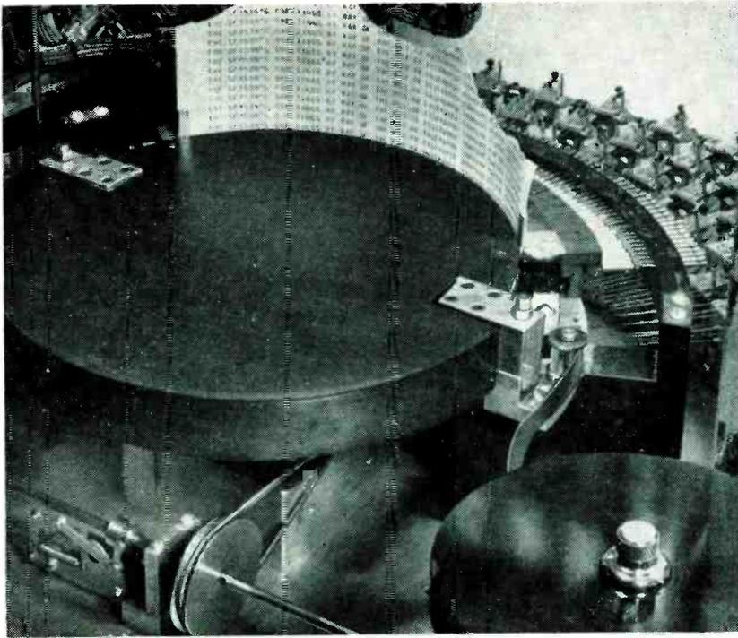
Eighty solenoid-controlled hammers, one for each column, strike type face through ink ribbon and paper to form letter impressions
