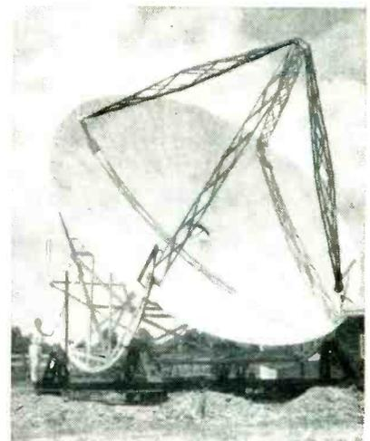
Parabolic receiving antenna used in moon reflection experiment
