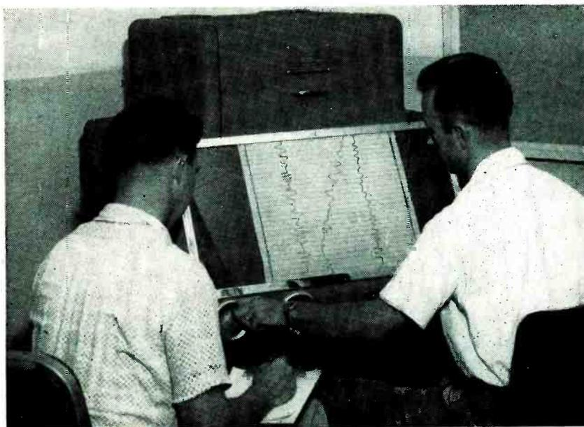
Semiautomatic machine scans photographic recordings of telemetered data. Points are read by manually positioning x and y cross hairs and reading coordinates on mechanical counters
