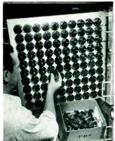
Pull-out drawers for aging tubes. Each drawer has 100 sockets. Operator is here loading one with type 6095's, which are the ruggedized equivalents of 6AQ5 pentodes
