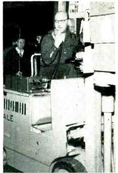
Two-way radio on lift truck
