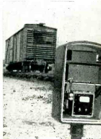
**OPERATOR** in freight-yard control tower (left) engages remote car-retarder when speed meter (right) warns that coupling speed is unsafe as . . .
