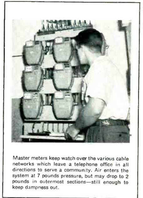
Master meters keep watch over the various cable networks which leave a telephone office in all directions to serve a community. Air enters the system at 7 pounds pressure, but may drop to 2 pounds in outermost sections—still enough to keep dampness out.
