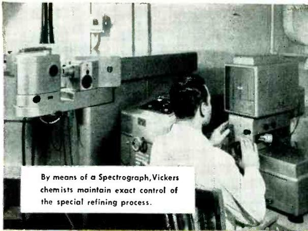
By means of a Spectrograph, Vickers chemists maintain exact control of the special refining process.
