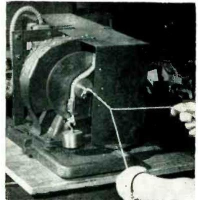
Method of using modified tapping machine for twisting leads together
