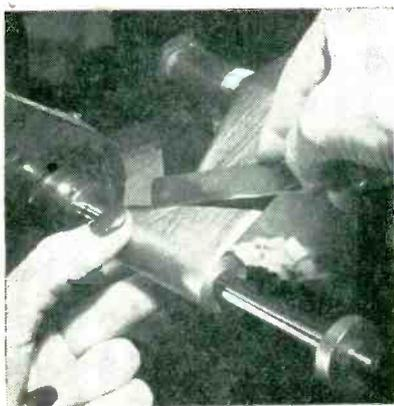
Cutting foil and paper layers of finished capacitor with knife made from hacksaw blade
