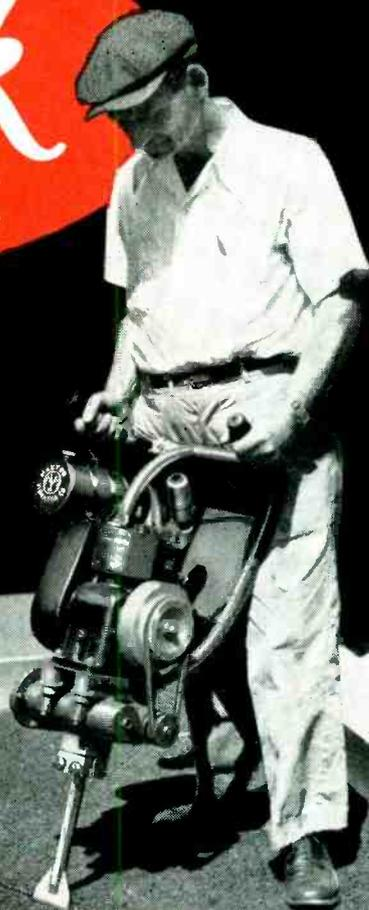
Everlock washers give added dependability to the Master Tamper, manufactured by the Master Vibrator Company, being used here as an asphalt cutter
