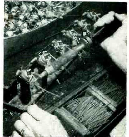
Six-unit holding fixture speeds subassembly work on television receiver controls by providing best work angle
