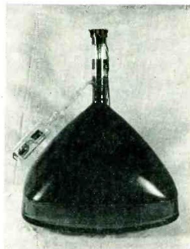
Method of installing ionization gage on picture tube for correlating gas ratio measurements with gas pressure in tube
