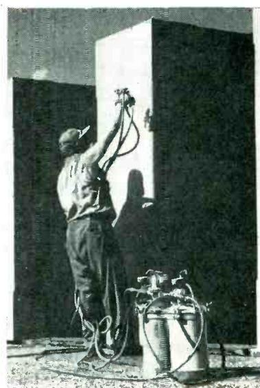
Spraying concrete blocks for cosmotron with dust-preventing resin. Preliminary tests indicate the solution also has waterproofing value
