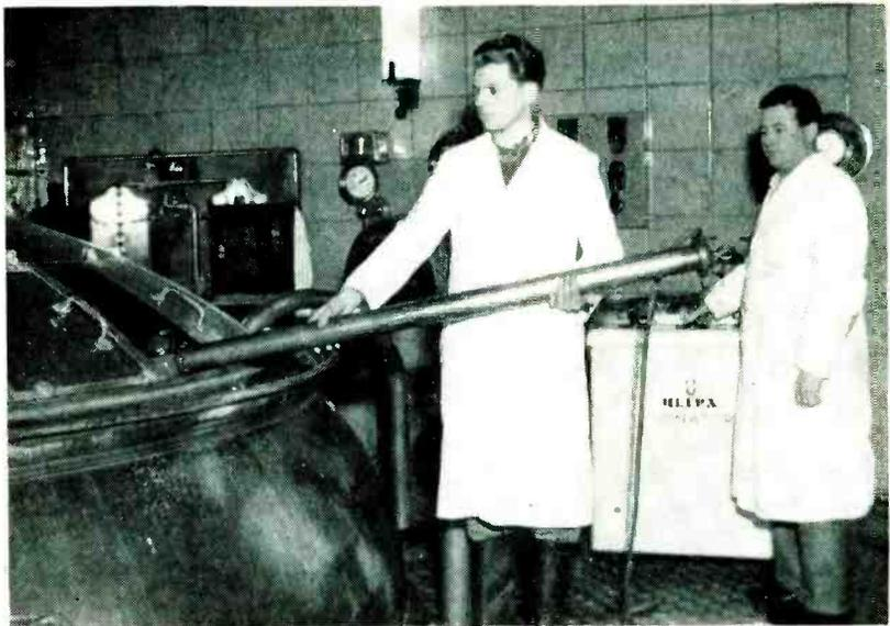
Brewer lowers copper-sheathed ultrasonic transducer into beer vat while assistant prepares to switch on 1-mc generator
