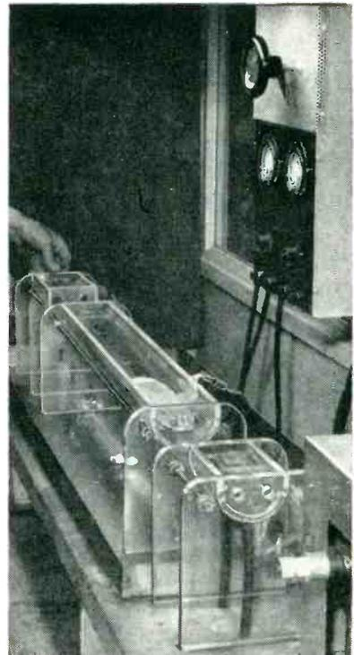
Reel of unplated wire is at left. Take-up reel for silver-plated wire is at right, on shaft of motor housed in metal box
