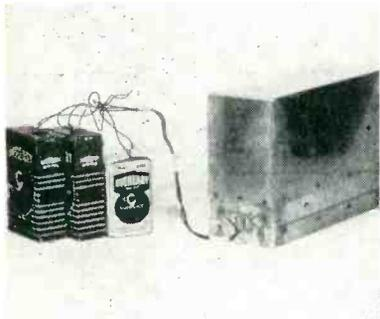
Test oscillator completely shielded but with batteries and supply leads external
