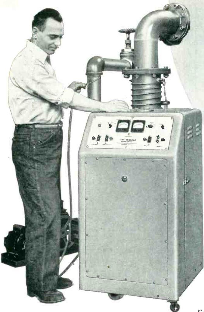
*Consolidated Engineering Leak Detector, Model 24-101A (above) is a simplified mass spectrometer sensitive to minute traces of helium. It can be used with either the probe or envelope method. The self-contained unit includes mechanical and diffusion pump; and all necessary controls and instruments.*
