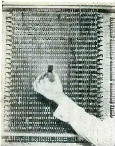
FIG. 1—Magnetic toroid and coils are sealed in plastic. Background is memory matrix using the toroids
