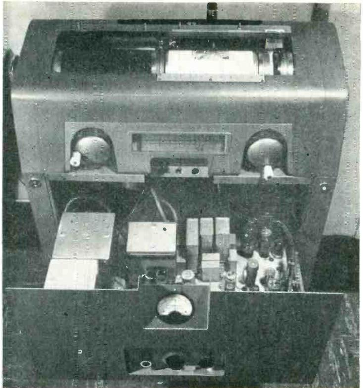
Machine with chassis drawer open. Pointers on slide-rule dial, controlled by hand wheels show side-border limits to which machine has been set. High-voltage power supply for stencil-cutting spark is on a lower chassis along with electrode feed circuit
