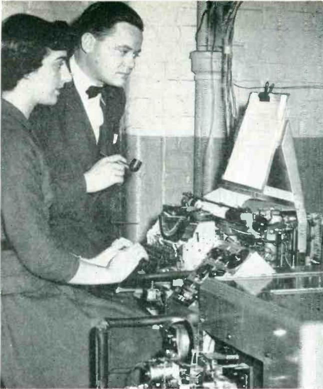
Electronic photocomposing machine used to make negatives from which an entire book, "The Wonderful World of Insects", was recently produced. Housing of this developmental model has been removed to show mechanism.
