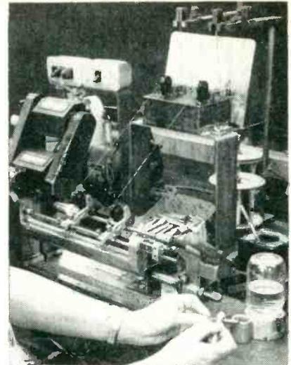
Dual-mandrel coil-winding setup in which wire is run through rectangular tank filled with solvent just before being wound on the coils. Cement dispenser is at lower right, with electrically heated wax pot behind it
