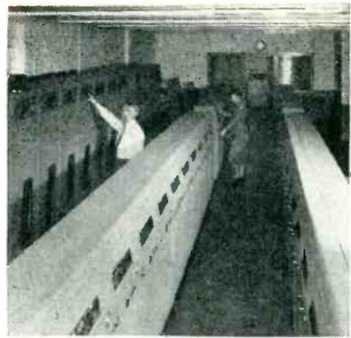
Manual forwarding units are at left, and cross-office units and multiple call processing equipment are at center and right in this view of the teletypewriter switching center
