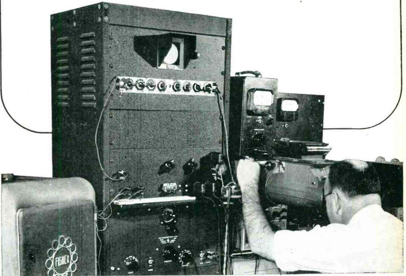
This Armco laboratory technician is measuring the performance of 4-mil thick Armco Electrical Steel under a new test condition. To find out what this steel will do in actual service, the test sample used is a typical magnetic amplifier core. Moreover this core is heated to 105 degrees C and held at this temperature to approximate one of the extremes of working conditions.
