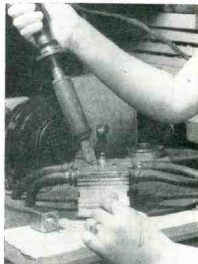
Production setup for keeping discriminator cool while making hermetic solder seal
