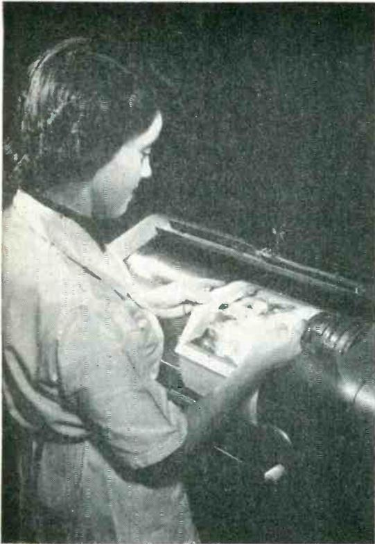
Placing original copy on Roco stencil machine. Stencil is rolled around left-hand cylinder. Adjustable cam disks at right, acting on snap-action switches, can be set to crop top and bottom of copy
